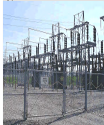
Exhibit 2-19 Typical 230 kV Substation
