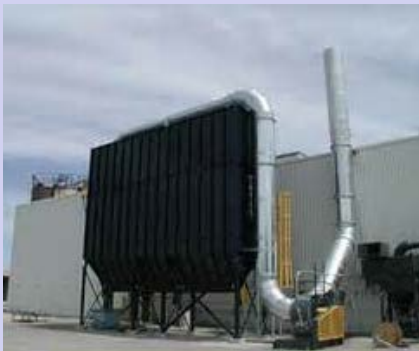
Metal Dust Collection System
