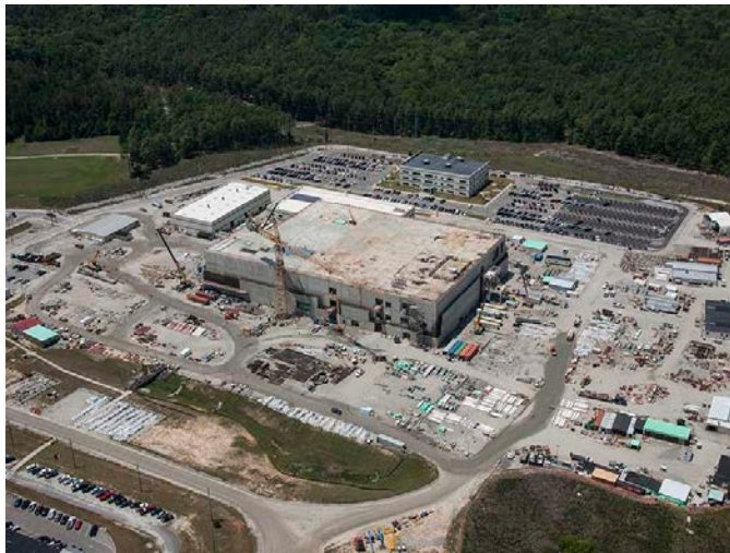
Mixed Oxide Fuel Processing Facility
