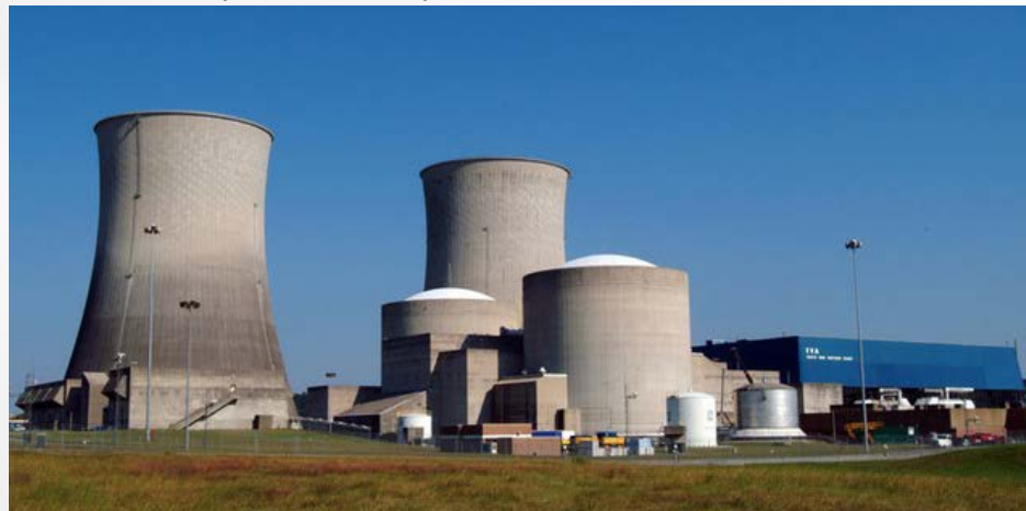
Watts Bar Nuclear Plant Spring City, TN
