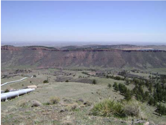
Chimney Hollow Valley and Flatiron Penstock
