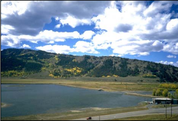
Existing Windy Gap Reservoir, Grand County, Colorado
