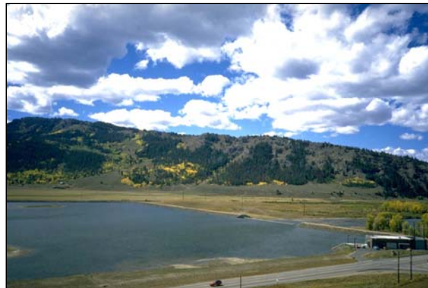
Existing Windy Gap Reservoir, Grand County, Colorado
