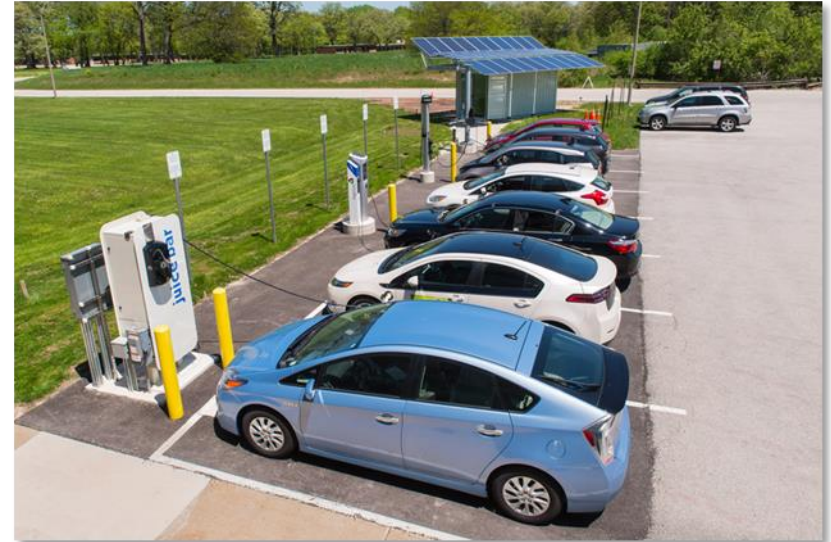
ANL EV Charging Station Infrastructure interfaced with Energy Storage and Solar Generation System
