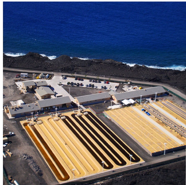
Aerial view of Cellana’s demonstration facility in Kona, Hawaii. Photo courtesy of Cellana, Inc.
