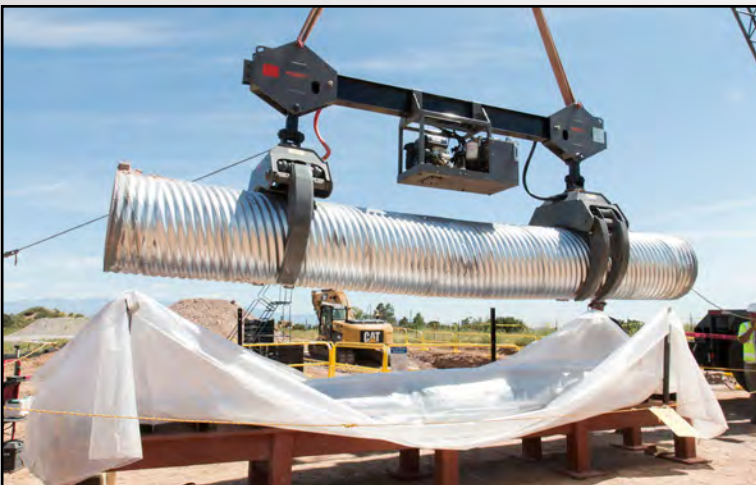
The crew places a demonstration CMP on the work table to be wrapped.
