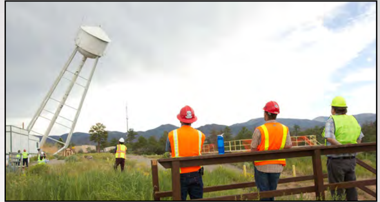
Workers watch while a water tower at TA-21 is brought down on Aug. 18.
