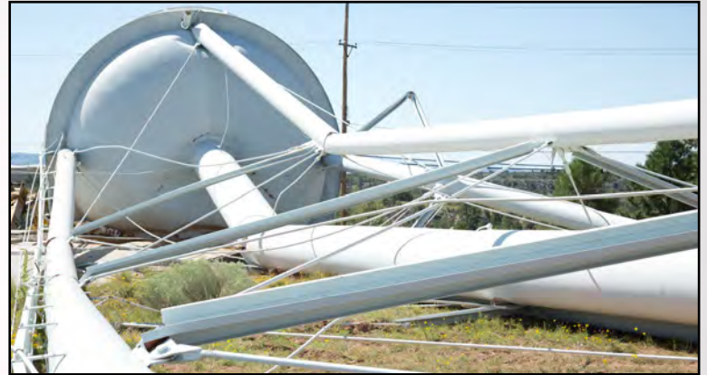
The towers will be dismantled and scrap material will be hauled to Albuquerque
