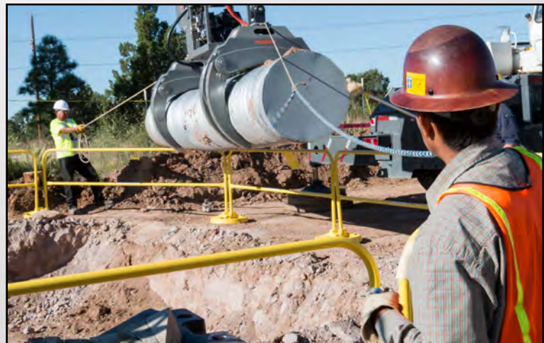
Two crew members help guide the rig by operating ropes called taglines.
