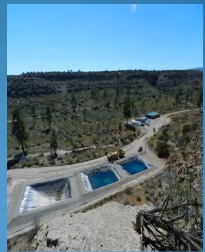
Basins for storing treated groundwater.
