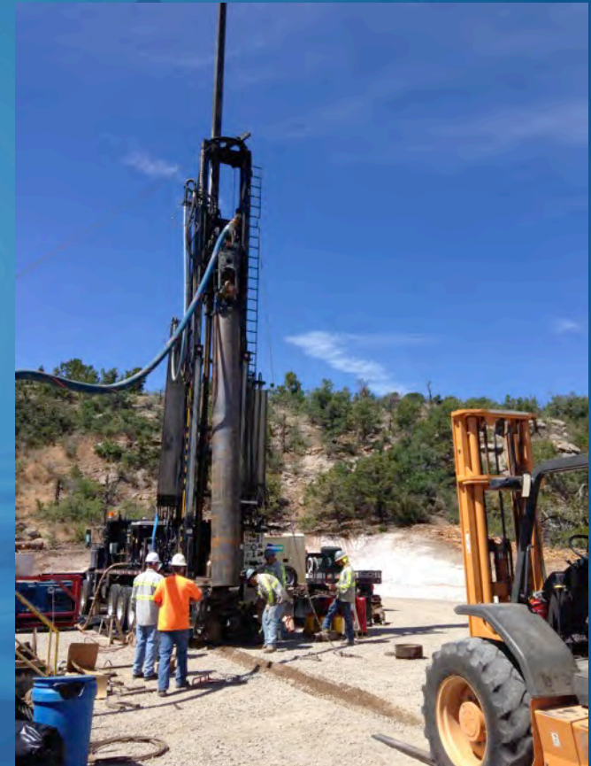
Drilling to install the CrEX-1 extraction well began on July 4.
