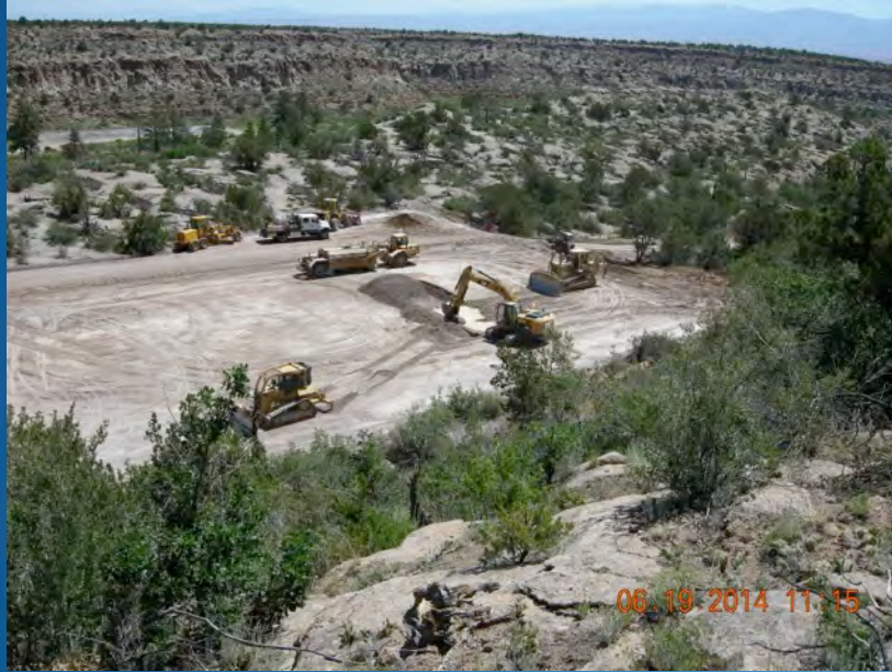
Constructing the pad for the CrEx-1 extraction well
