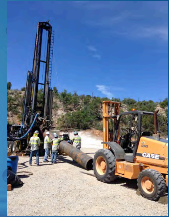
Drilling on the CrEX-1 extraction well began on July 4, 2014 and completed in early September.
