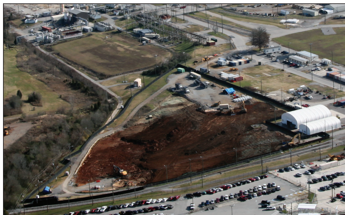
K-1070-B during remediation
