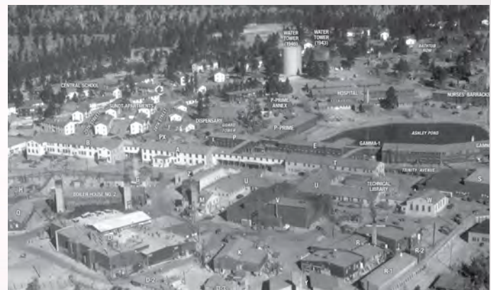
Former TA-1 was the core of the original Laboratory during the Manhattan Project and early Cold War era. It was decontaminated and demolished in stages until the entire site was given to Los Alamos County or sold to private interests.
