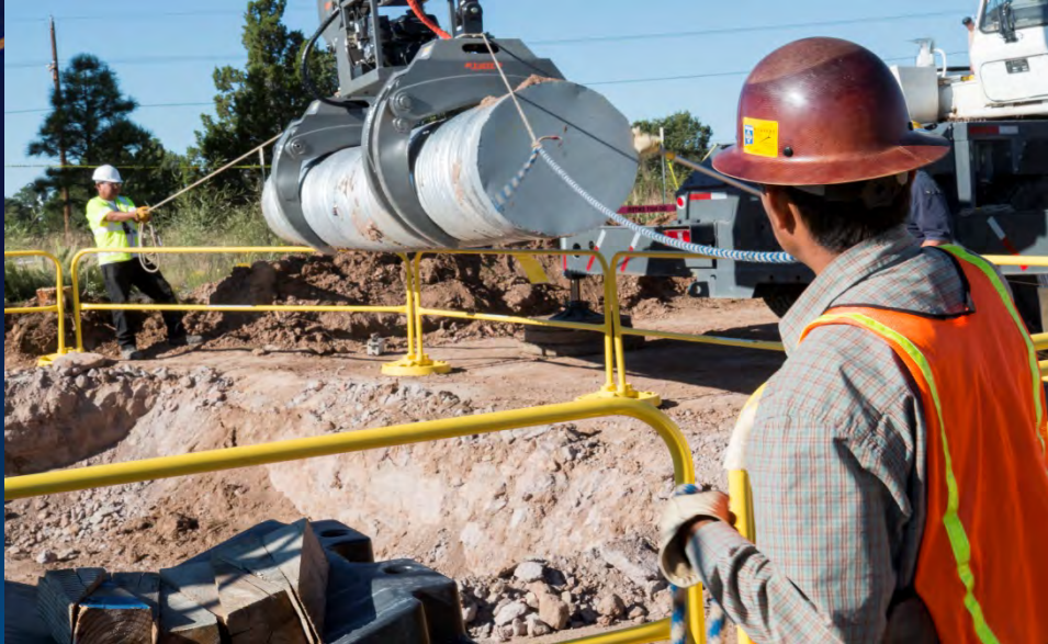
Crew members operate tag lines to help guide a demonstration of corrugated metal pipe (CMP) retrieval from the CMP array onto a large metal table to be surveyed and wrapped.
