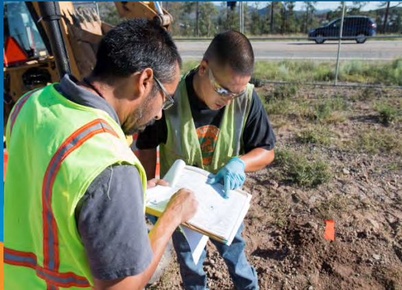
A cleanup project is underway at TA-61, located along the truck route near the county landfill.
