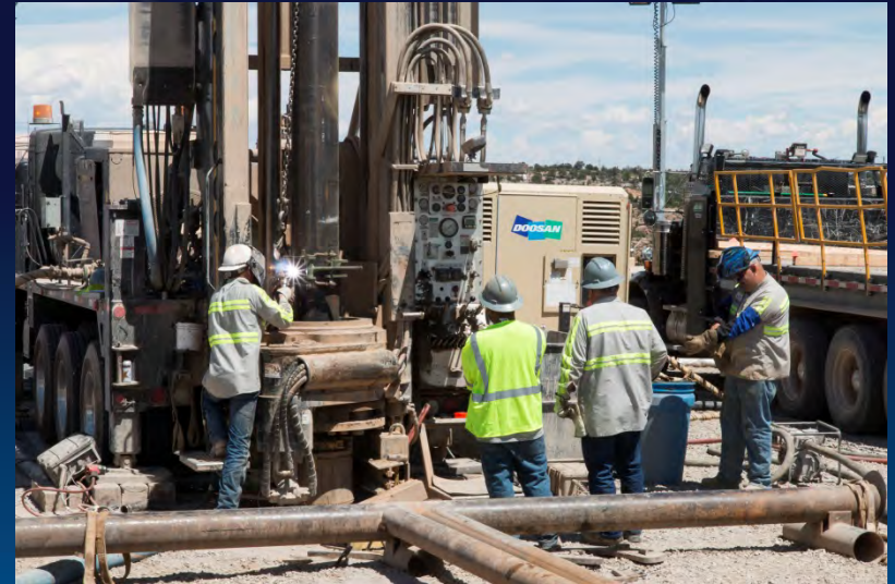
A crew prepares for drilling to begin for CrCH-1 (chromium core hole 1) in Mortandad Canyon in support of chromium remediation.
