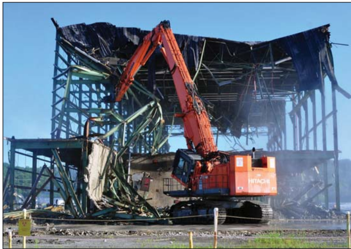
Demolition of K-31 nears completion in June.
