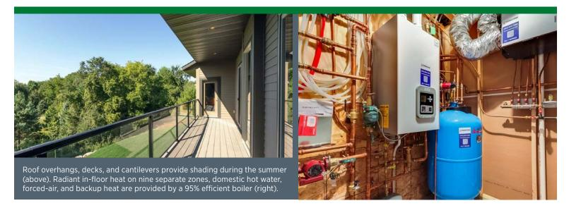
The home's heating, ventilating, and air-conditioning (HVAC) system is based on radiant in-floor heat with nine separate zones (which also provide thermal mass with tile for passive solar). It has a 110,000-Btu, 95% efficient boiler that provides domestic hot water and in-floor heat. A forced-air, 95% efficient, two-stage, fully modulating furnace on two electronic zones provides backup heat.
