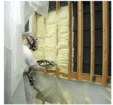
(Left) Contractors are installing the 2×4 framing on the existing siding of Test House 2. (Above) The spray foam is being installed within the new framing.
