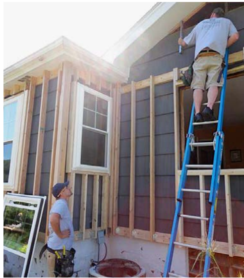
(Left) Contractors are installing the 2×4 framing on the existing siding of Test House 2. (Above) The spray foam is being installed within the new framing.
