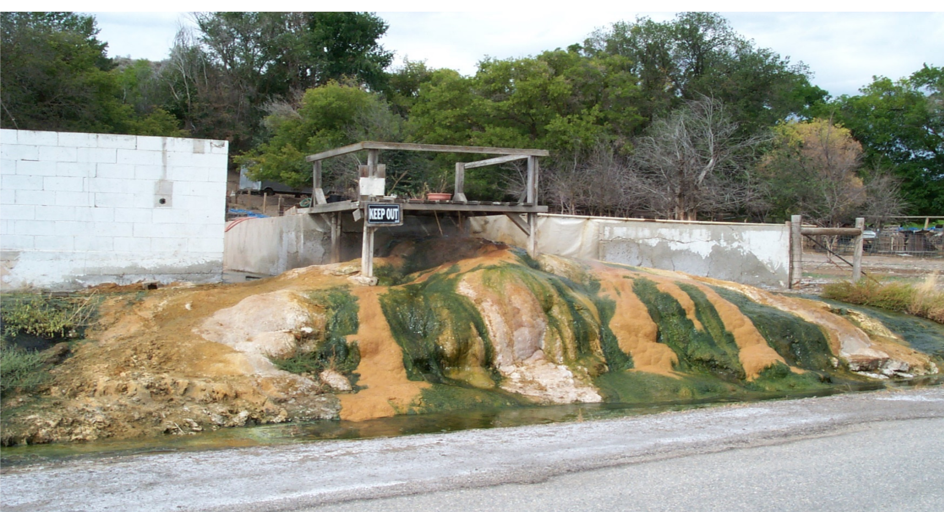
Figure 3. Dilapidated structures remaining from the Squaw Hot Springs, Northern Cache Valley, Idaho. This spring is near the southern extent of the Preston Geothermal Prospect. The springs discharge 73 °C water and a well drilled on the property yielded 84 °C water (Mitchell, 1976). RTE results predict a reservoir temperature of 179 °C (Wood et al., 2015).
