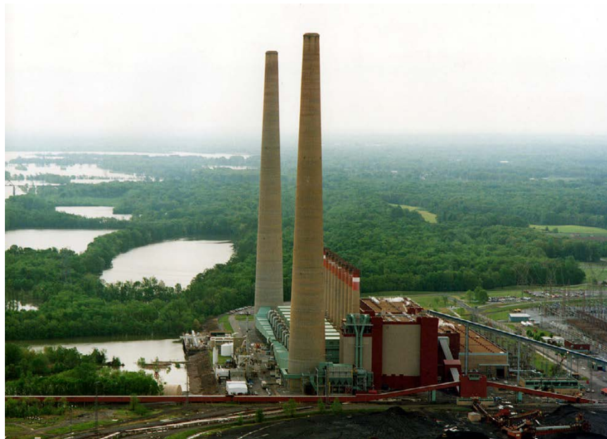
Figure 4-2. Aerial view of Shawnee Fossil Plant.
