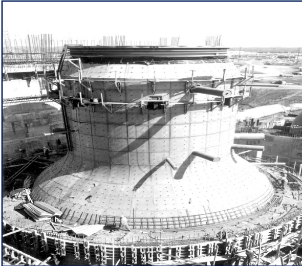
Oak Ridge Site. Construction of nuclear power reactor. (c. 1970)
