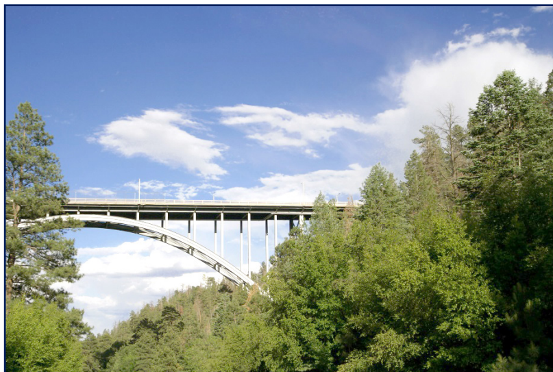
Los Alamos Canyon Bridge. Constructed in 1951, the Los Alamos Canyon Bridge is a historic structure and a main transportation route between Los Alamos and the laboratory.
