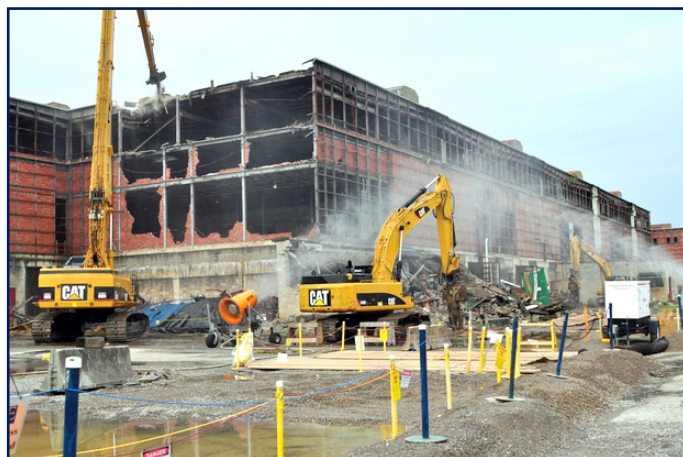
Oak Ridge Site. Demolition of the K-25 building.
