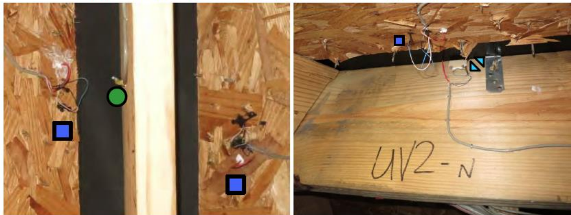
Figure 117: Ridge sheathing T/MCs and T/RH (L); ridge T/MC and wafer sensor (R)
