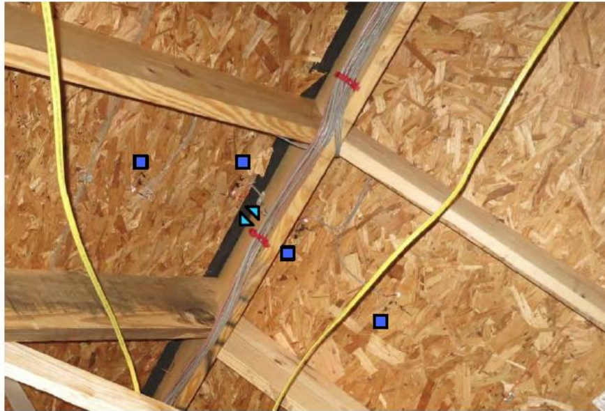
Figure 116: Typical ridge monitoring package, with sensors highlighted
