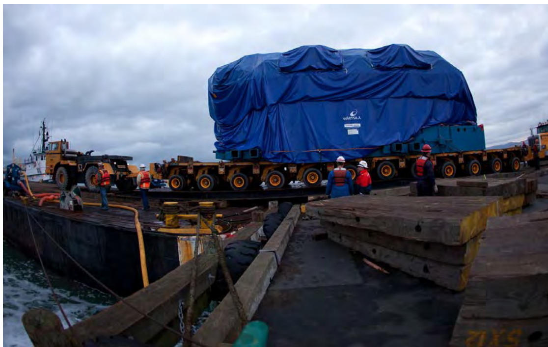
Photo courtesy of Bragg Crane & Rigging Co.
