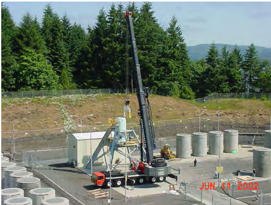
Photo courtesy of Trojan
