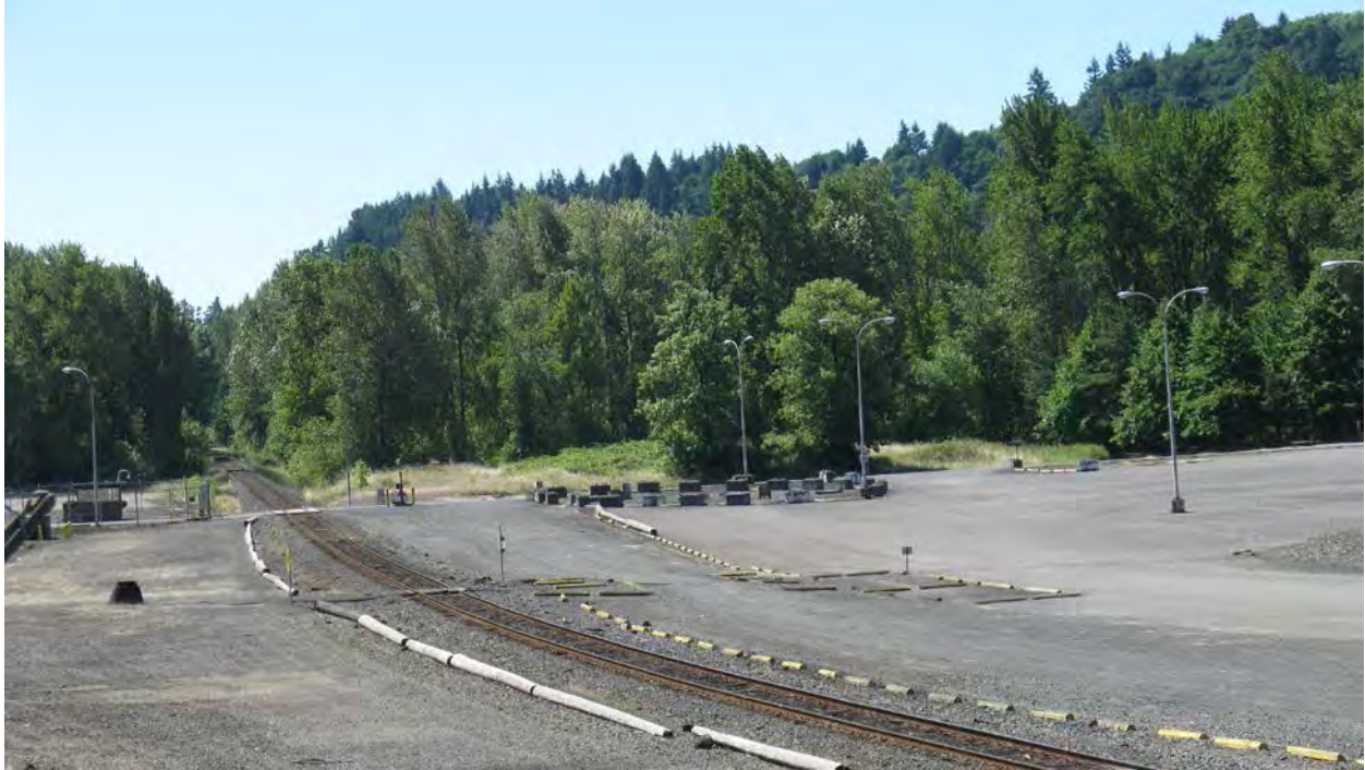
Figure 2-96. Portland and Western Railroad in the Vicinity of the Trojan Site
