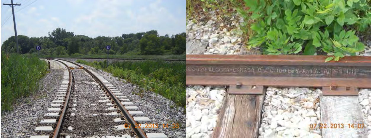
Figure B-17. Rebuilt Lead from the Zion Site to the Union Pacific Mainline
