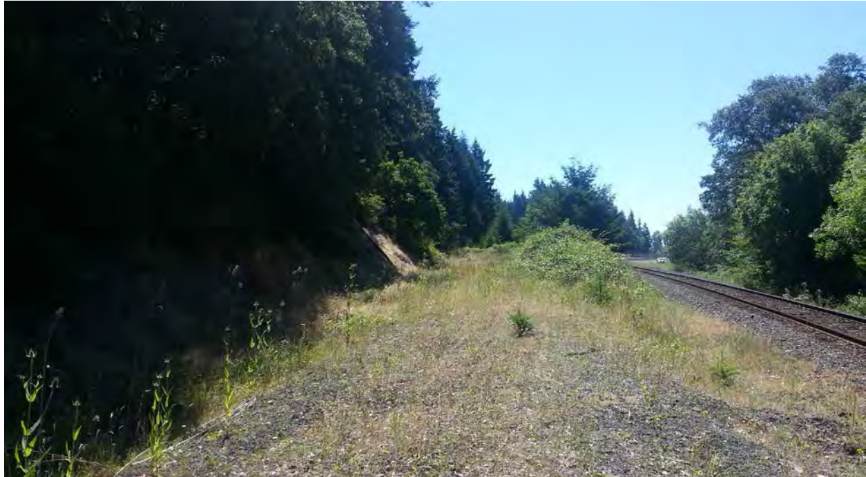
Figure 2-98. Former Trojan Rail Spur Railbed
