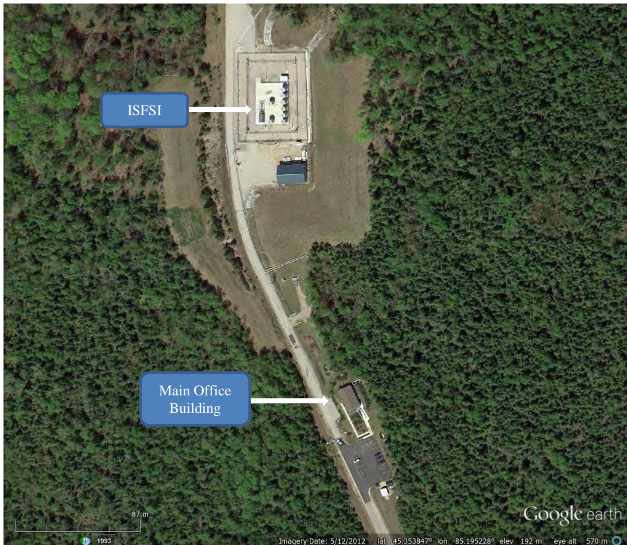
Figure B-3. Closer Satellite View of the ISFSI Pad and the Main Office Building at Big Rock Point (Google 2013)
