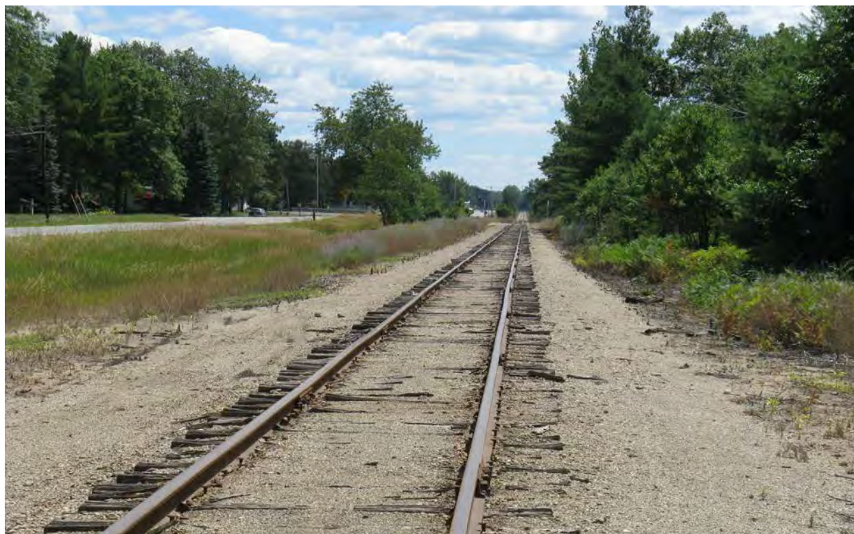
Figure 2-73. Condition of Rail Crossing in 2013 Used for Big Rock Point Reactor Pressure Vessel Transload (Looking South)
