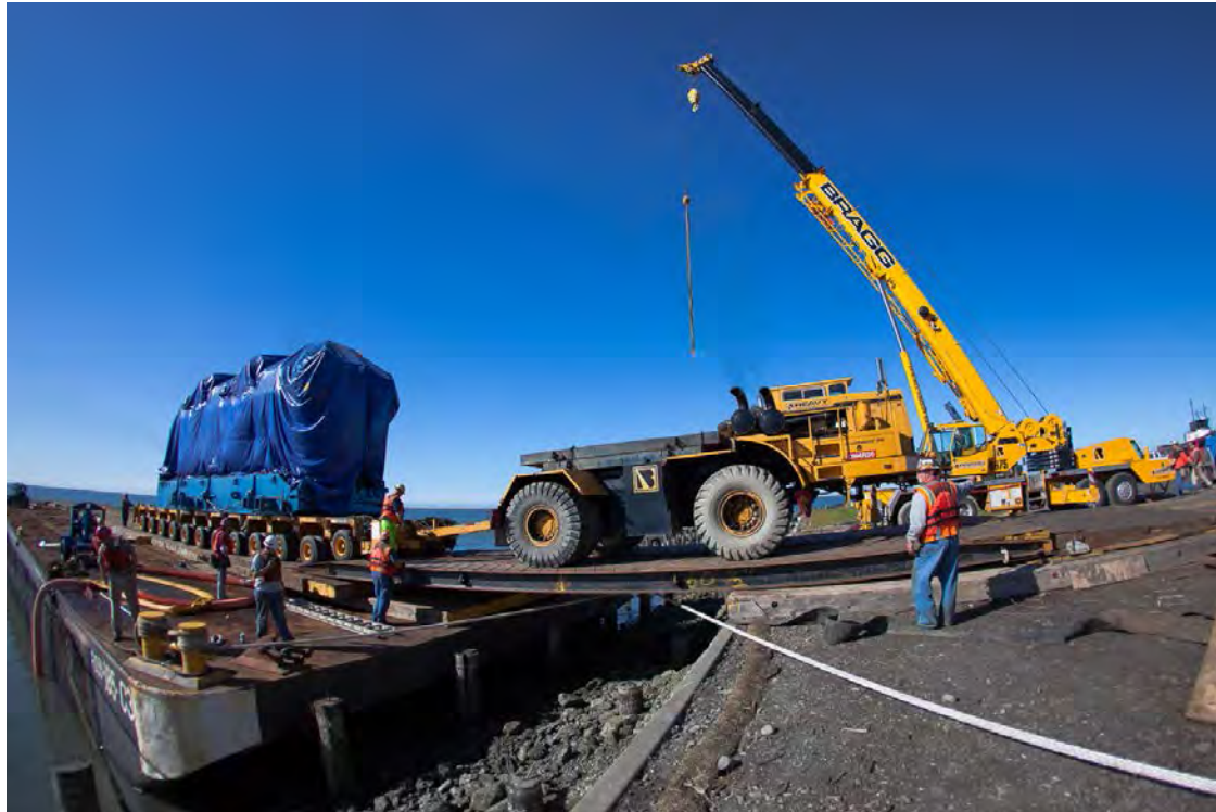
Photo courtesy of Bragg Crane & Rigging Co.
