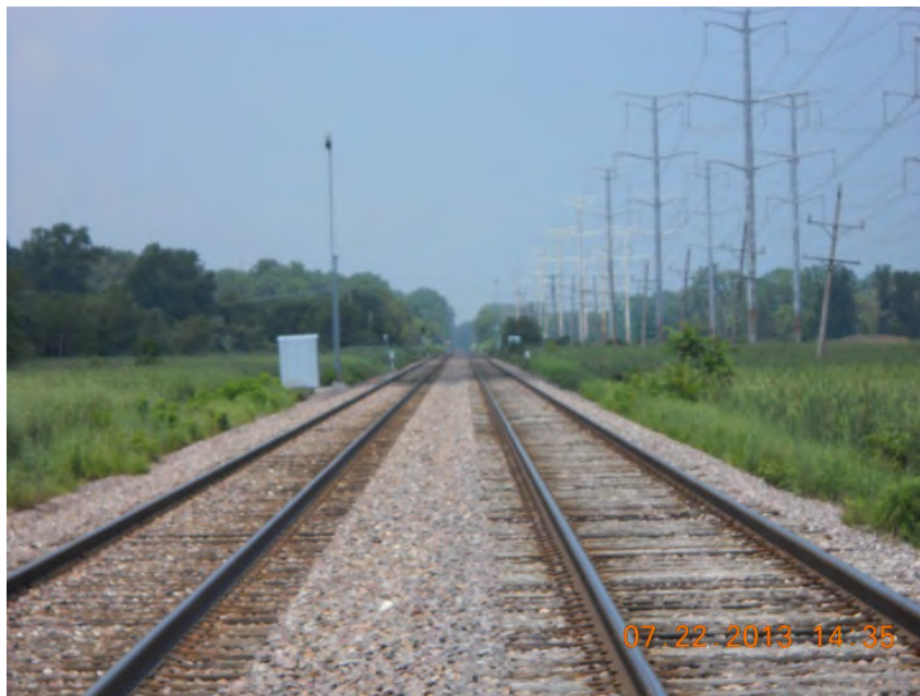
Figure B-16. Union Pacific Mainline at the Zion Site
