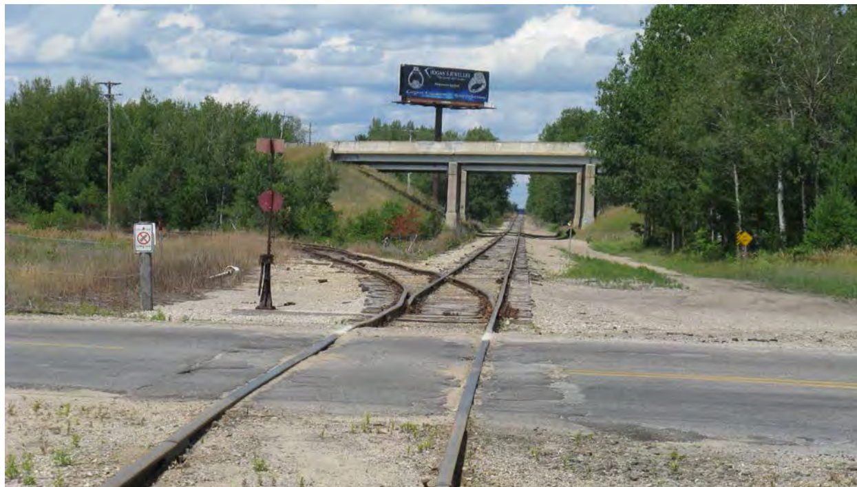
Figure 2-72. Condition of Rail Crossing in 2013 Used for Big Rock Point Reactor Pressure Vessel Transload (Looking North)
