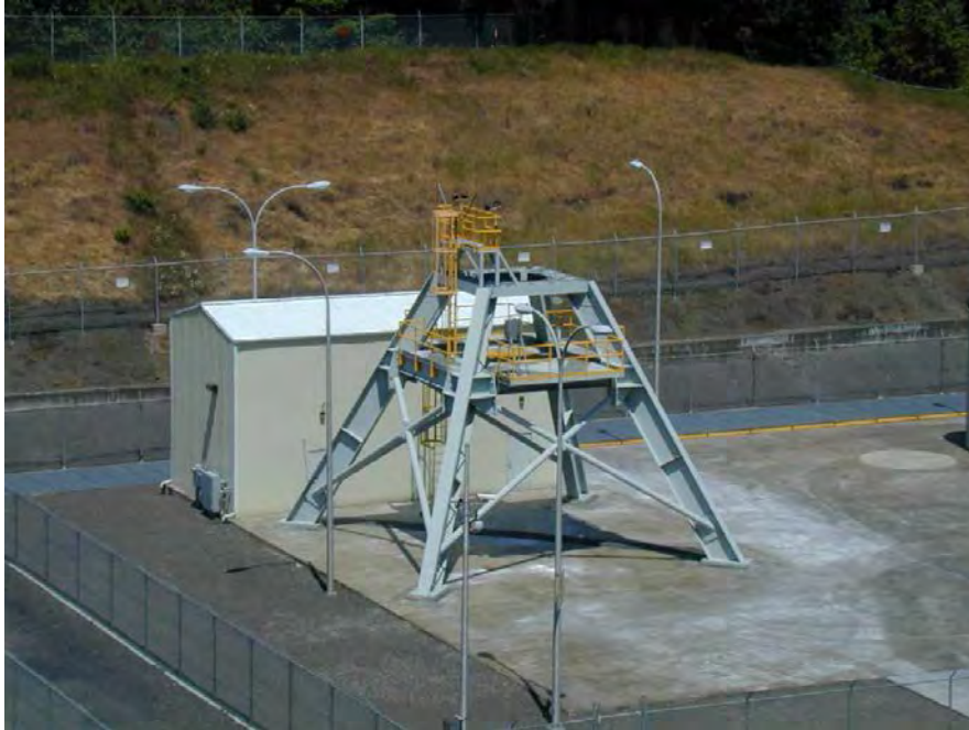
Photo courtesy of Trojan
