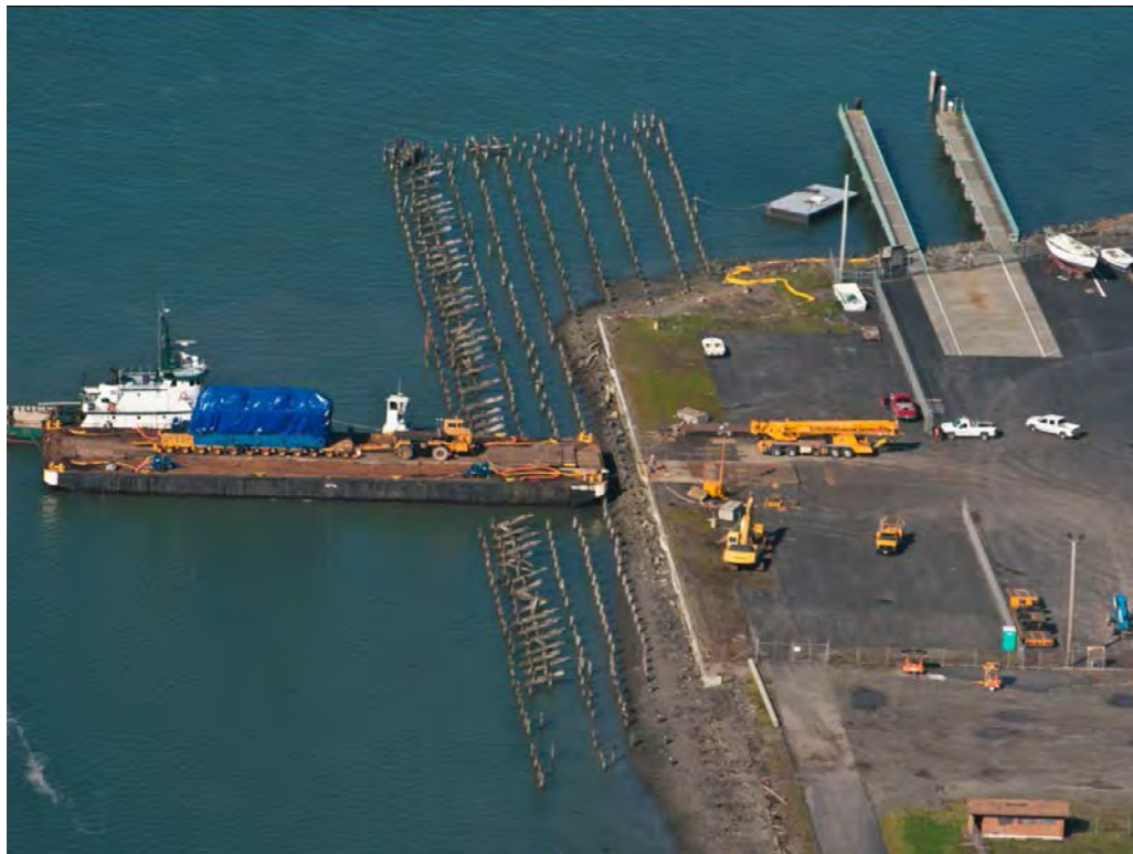
Photo courtesy of Bragg Crane & Rigging Co.
