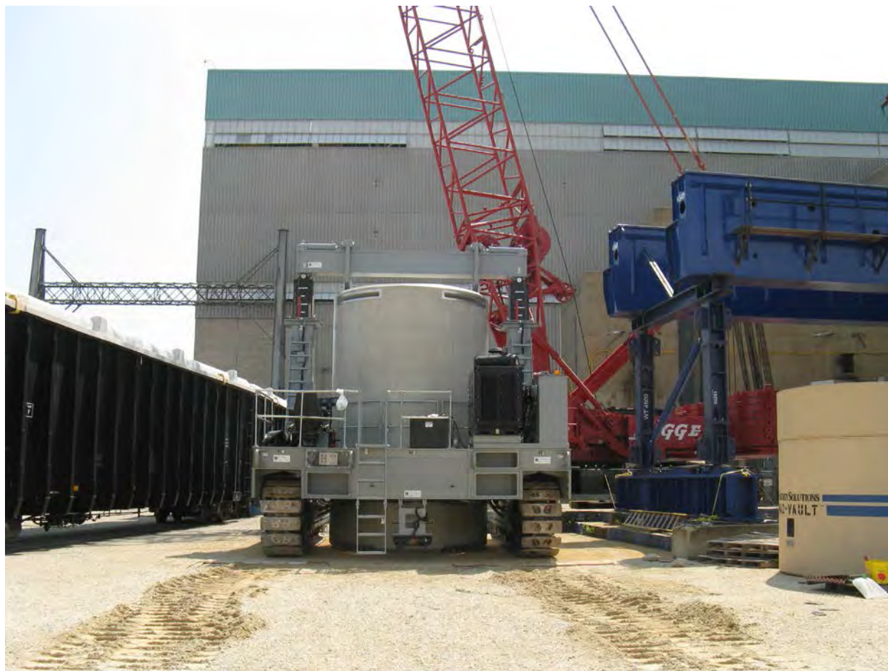
Figure 2-125. Transporter Used to Move Vertical Concrete Storage Casks
