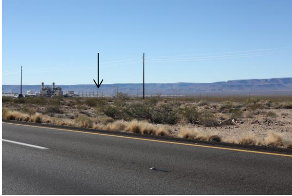
View of proposed project facilities, from I-40 approx. .65 miles northeast of Project location (arrow).
