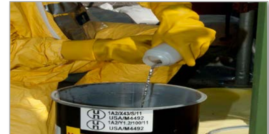
Mercury removed from storm sewers at Y-12
