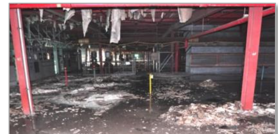
Inside of Building K-27 at ETTP
