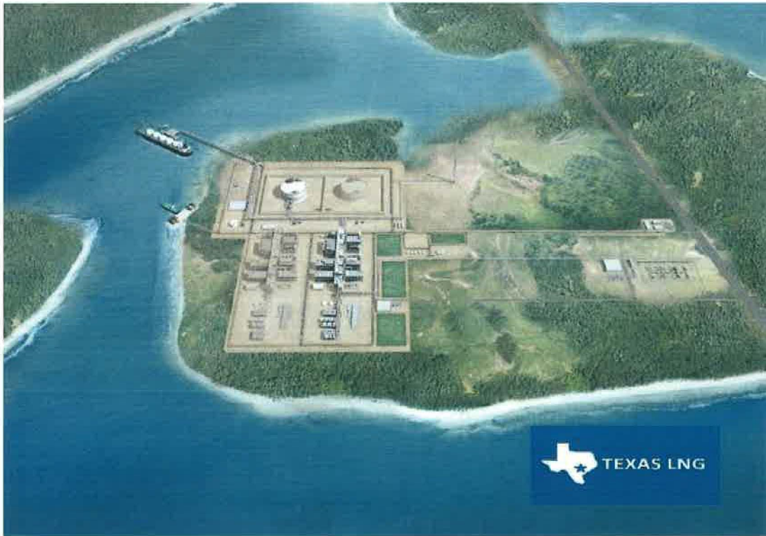
This image depicts Texas LNG’s planned liquefaction facilities.
