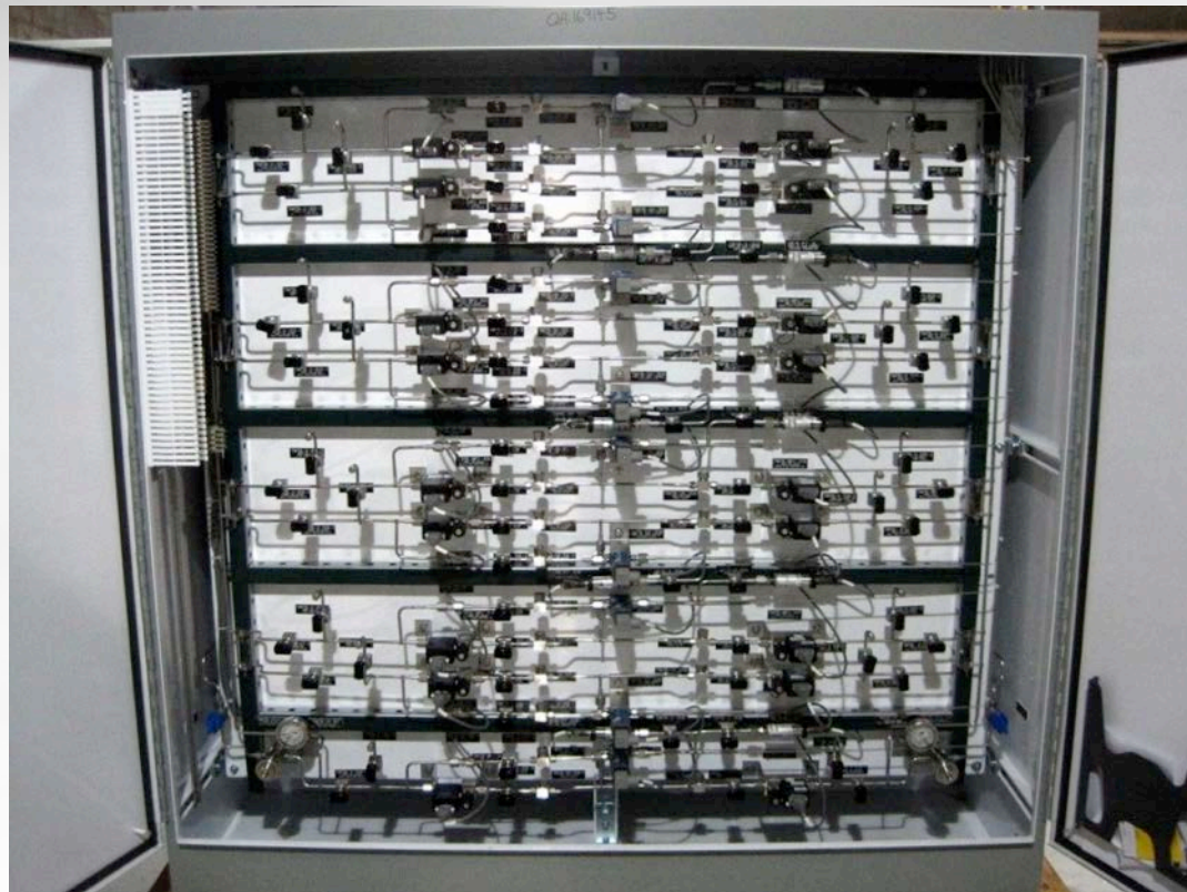
Temperature Control Gas Mass Flow Controller Cabinet
