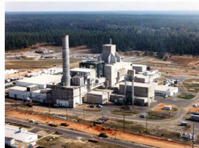
L Reactor at SRS
