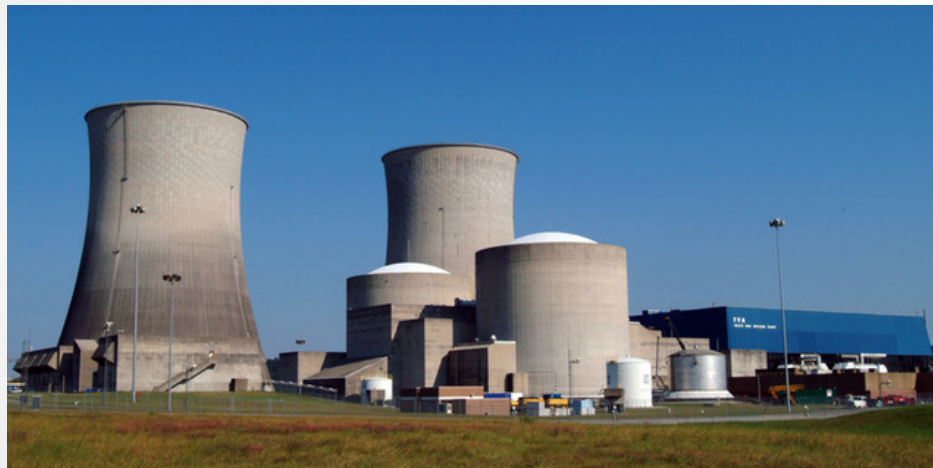
Watts Bar Nuclear Plant Spring City, TN
