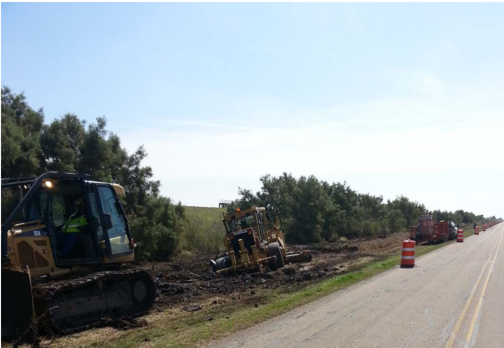
Photo 2. Grading activities along La Quinta Road.
