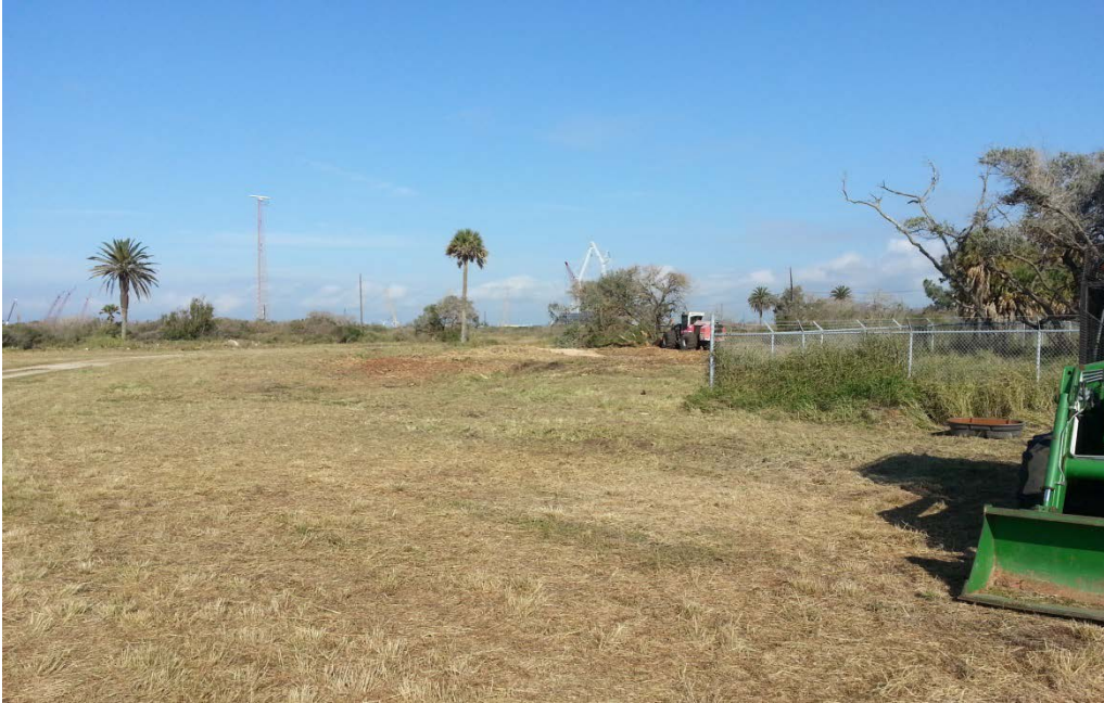
Photo 1. Site clearing at the CCL Terminal site.
