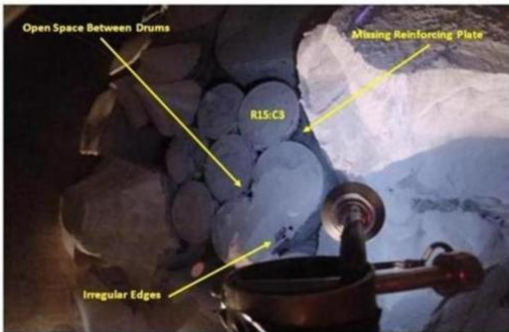
Figure 6-33: Missing Reinforcement Plate at R15:C3
