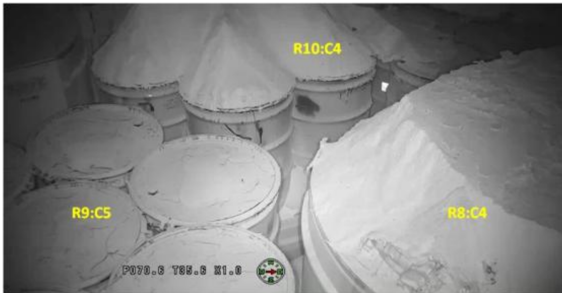
Figure 6-22: Damage at R9:C5 and R10:C4
