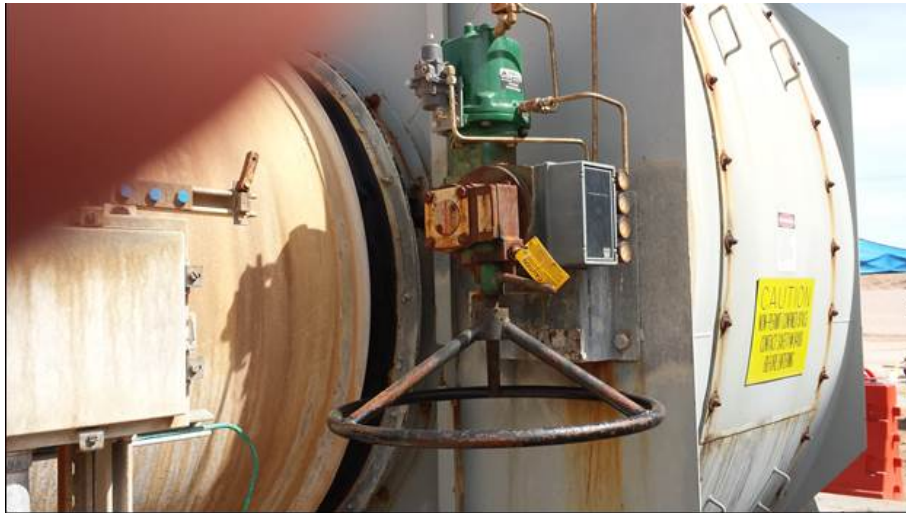
Figure 11: 860 Vortex Manual Hand Wheel
