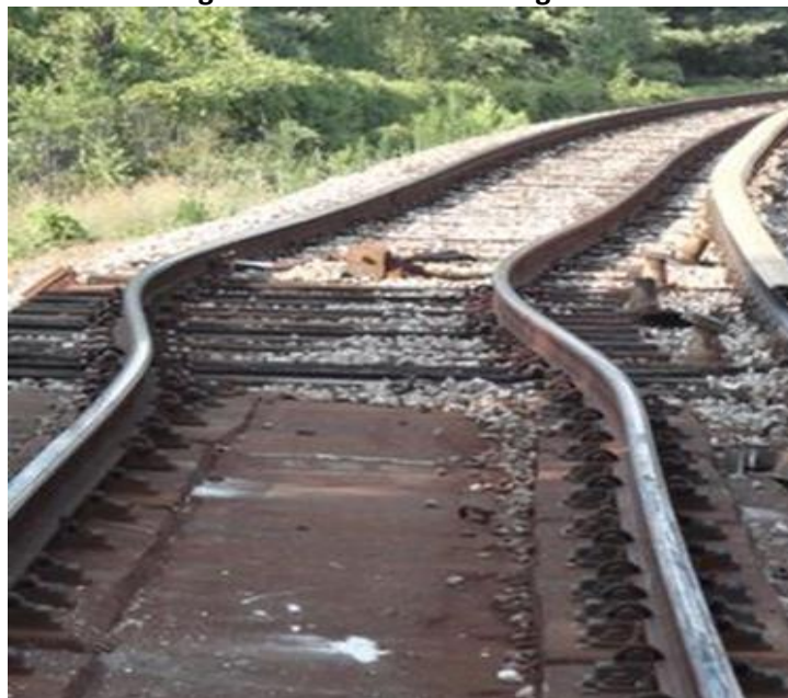
Figure 26: A Heat Kink along a Rail
