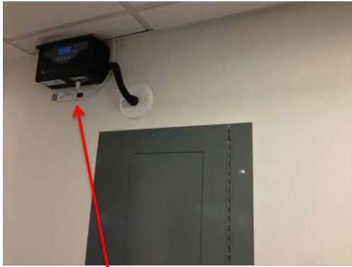
Panel Electrical Metering
