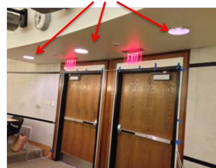
Lutron Lighting Control
