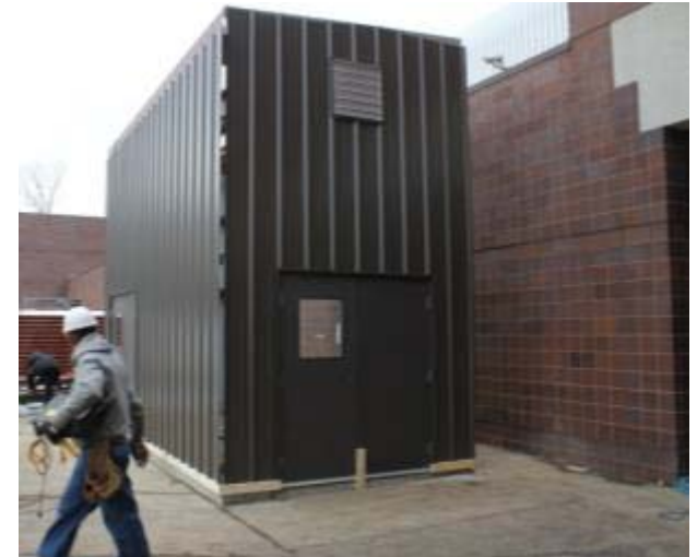
Biomass unloading building
