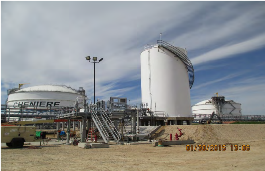
Condensate Storage & Send-Out System – LACT Skid (foreground) - Surface Coat applied.
