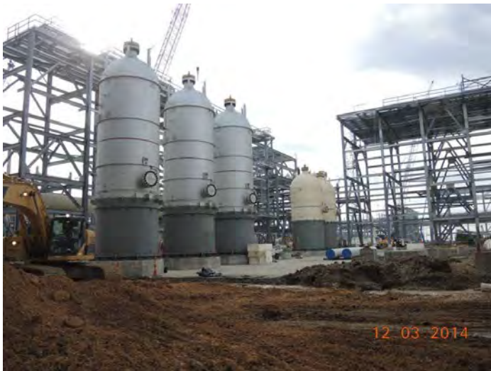
Train 3 Mercury Removal/Molecular Sieve Dehydrators
