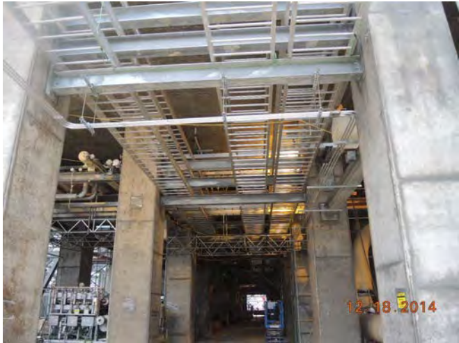
Train 2 Installing Cable Tray and Pipe under the Compressor Deck
