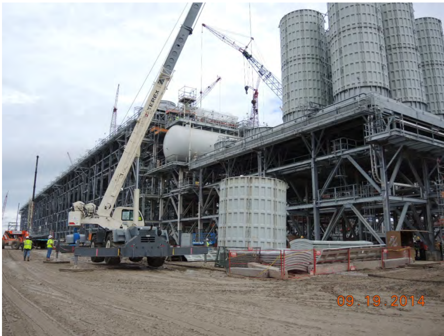
Train 1 Installing Plumes for Propane Subcoolers
