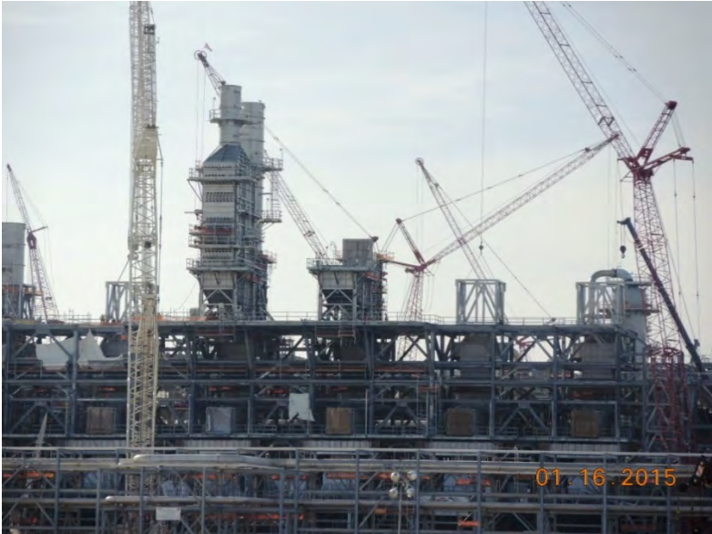
Train 1 Installed WHRU Elbow
