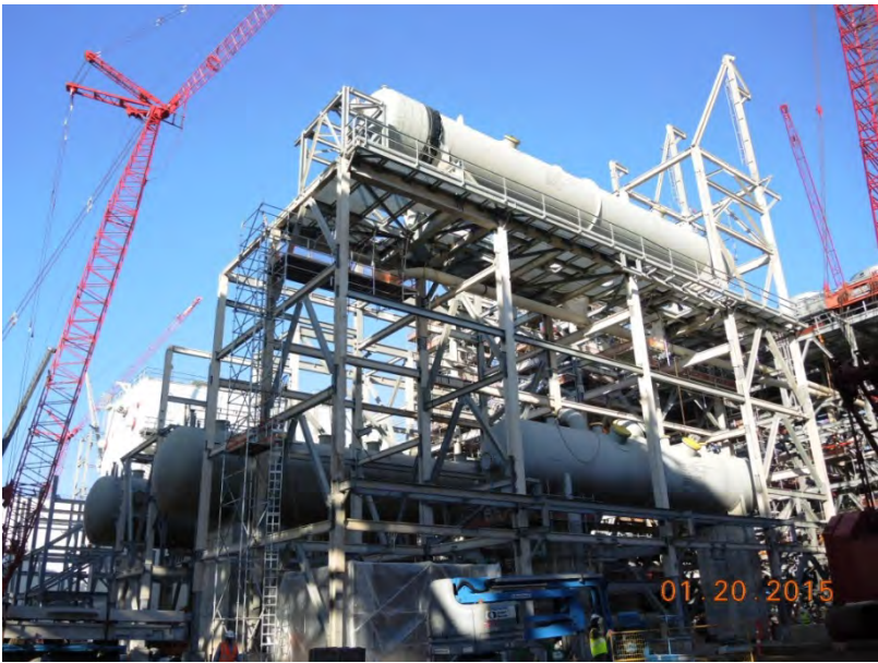
Train 2 Ethylene Surge Drum Installed
