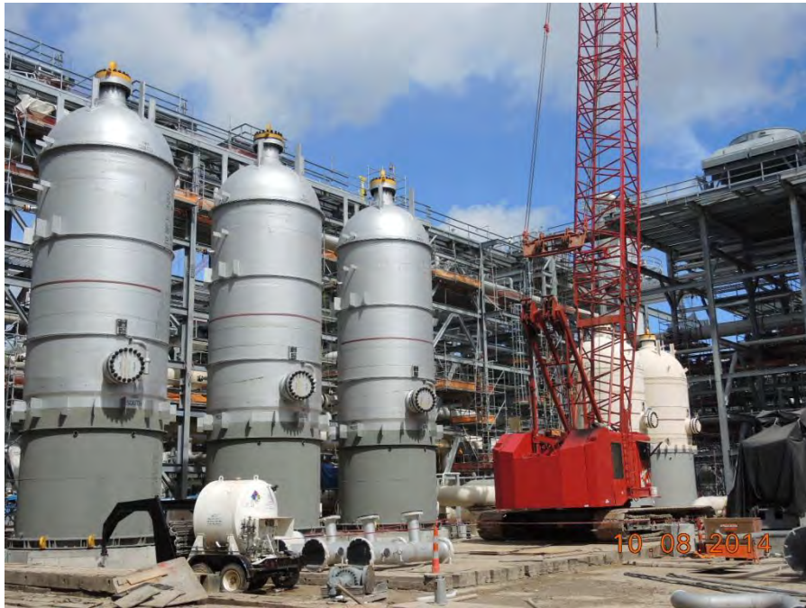
Train 2 Installed Molecular Sieve Dehydrators and Mercury Removal Beds
