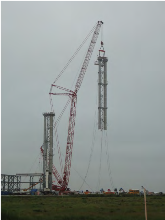
OSBL Stage 1 Setting top section of Wet Dry Gas Flare
