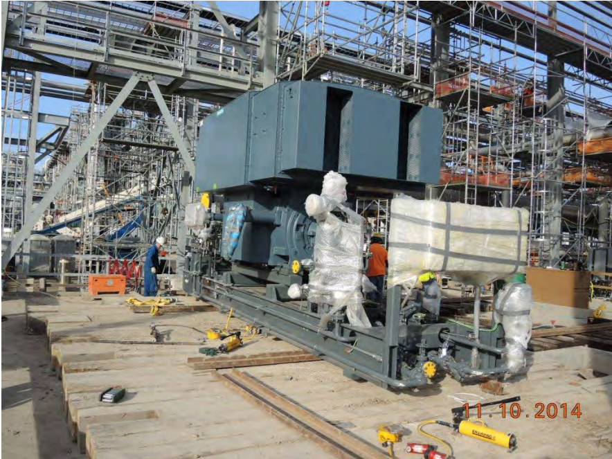
OSBL Stage 2 Setting BOG Compressor
