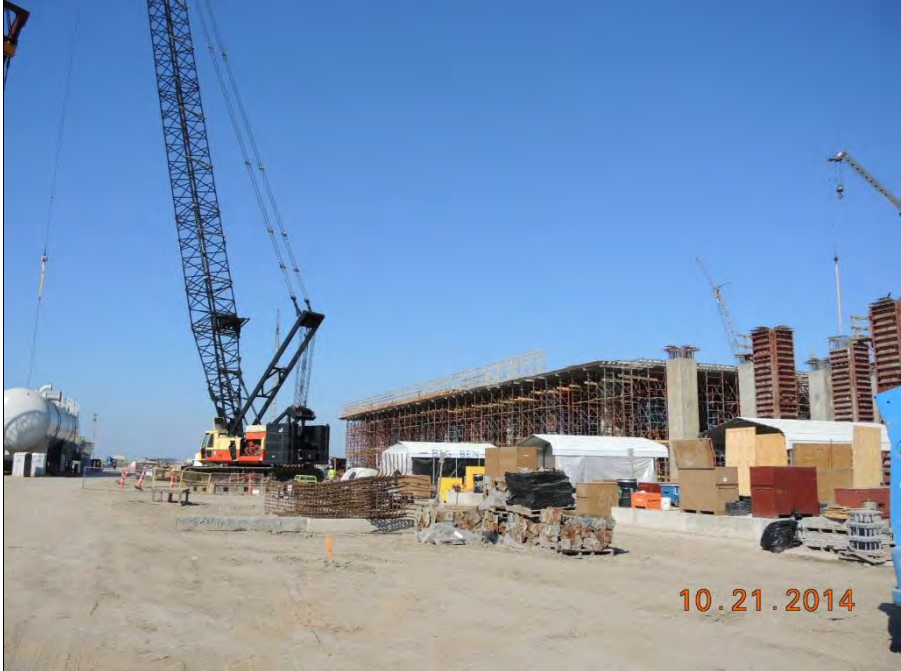
Train 4 Installing Rebar and Formwork on Compressor Deck
