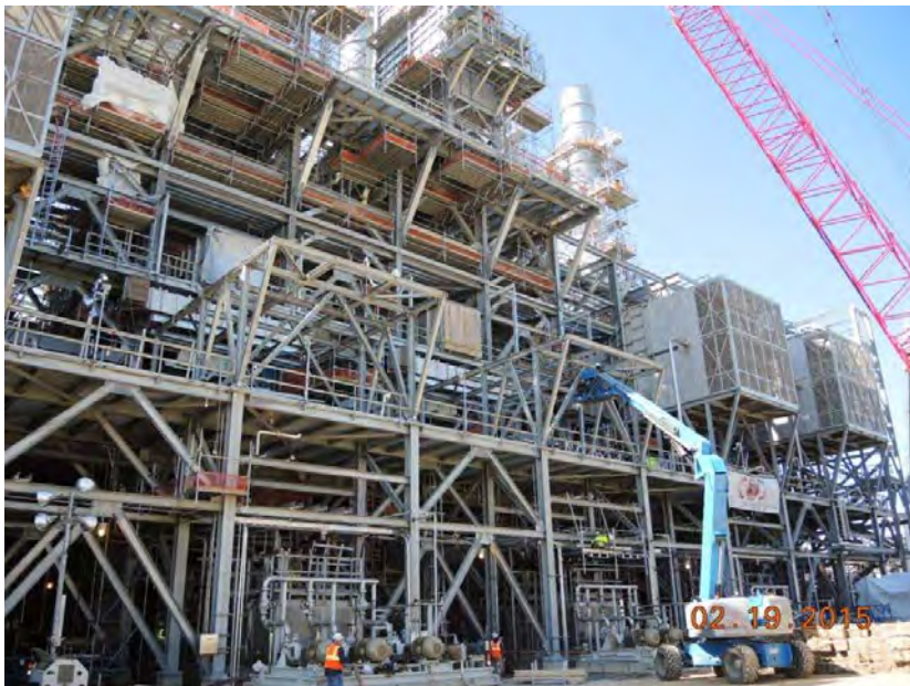
Train 1 Compressor Area - Installing bottom platform for ethylene filter houses.
