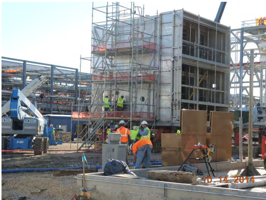
Train 1 Prefab of the Filter house
