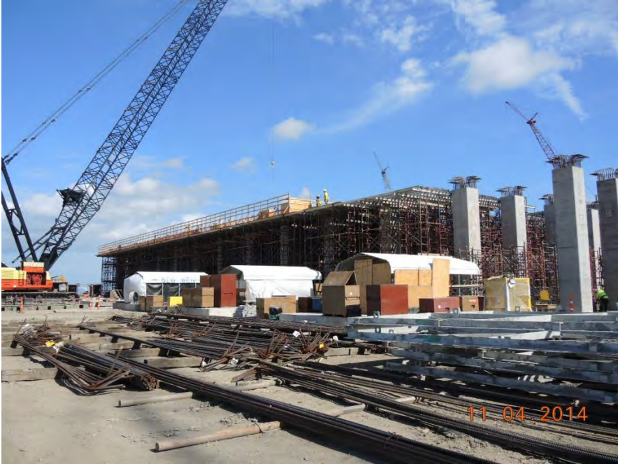
Train 4 Installing Table Top Rebar and Formwork
