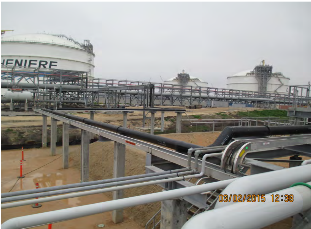
Black containment pipe (10") for 6" condensate line (pipe in pipe); has leak detection system.
