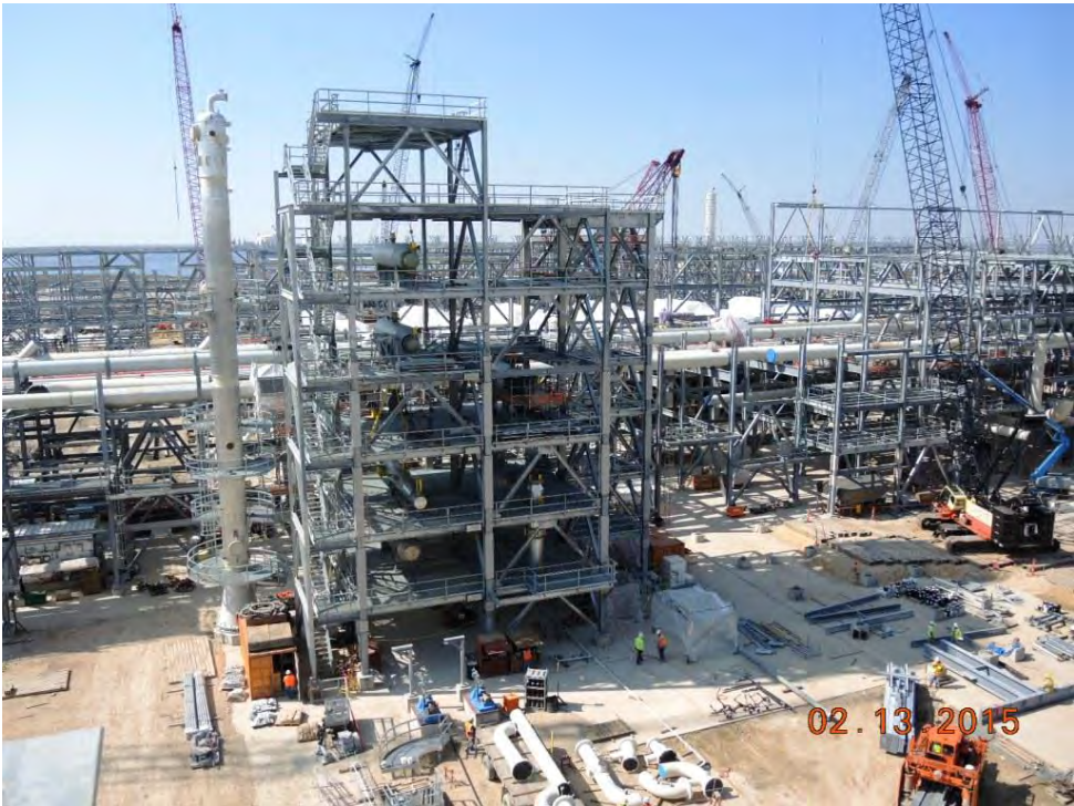
Train 3 Heavies Removal Area – Equipment & steel installation.
