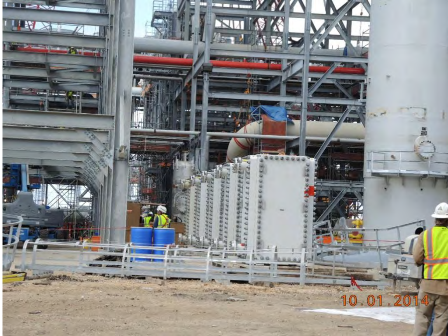
Train 2 Installed Lean Rich Solvent Heat Exchangers
