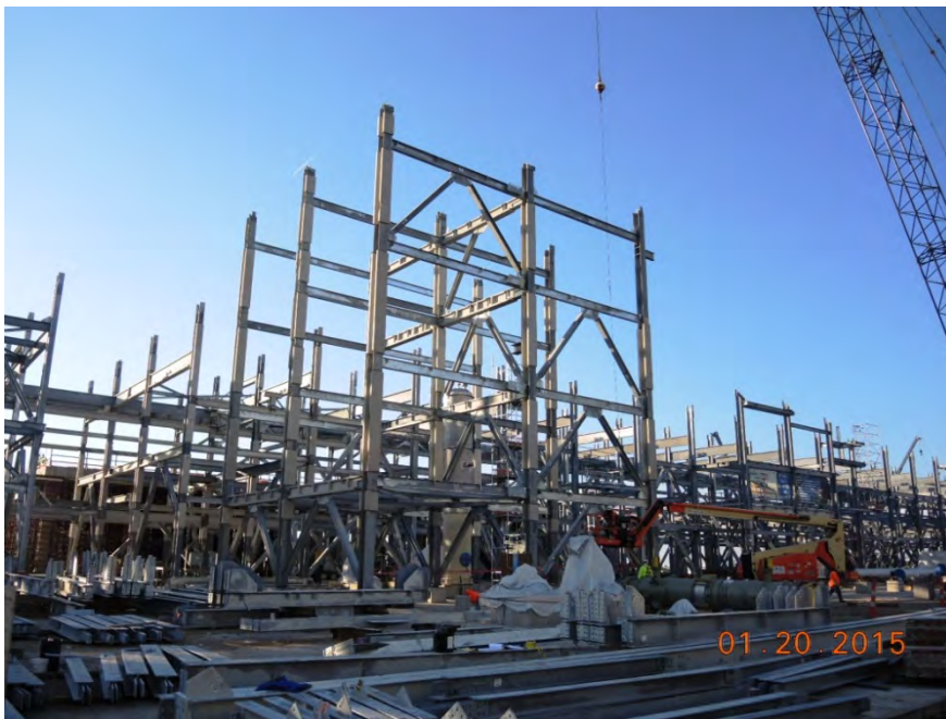
Train 4 Erecting Steel in Heavy Removals Area
