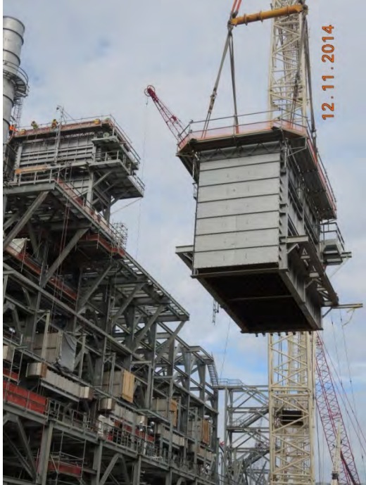
Train 1 Setting of the WHRU Upper Convection
