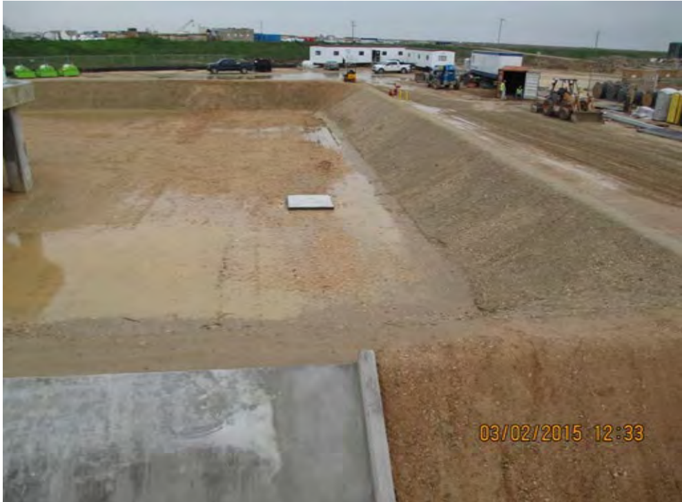
Completed Berm surrounding tank and LACT Skid.
