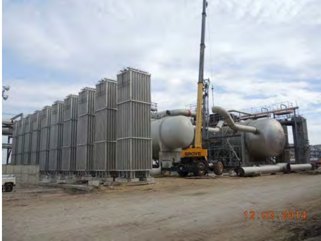
OSBL Stage 1 Flare Knockout Drum Pipe Installation
