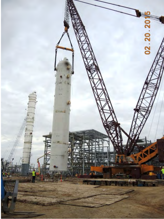
Train 4 Amine Regen Acid Gas Removal Area – Setting CO2 absorber.
