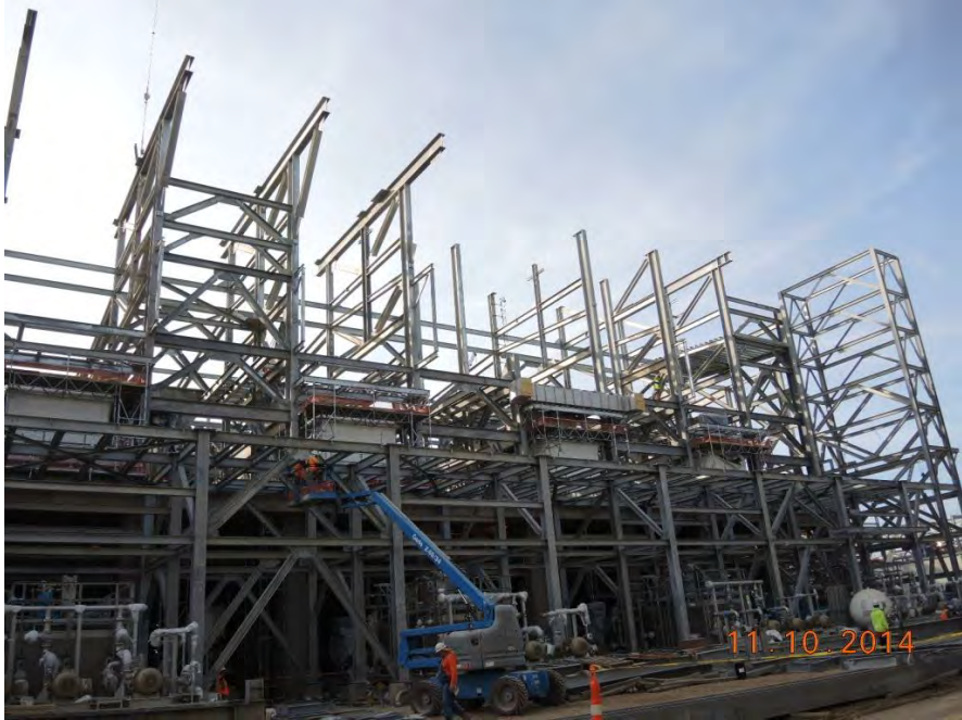
Train 2 Installing Inlet Ventilation Bull Horn
