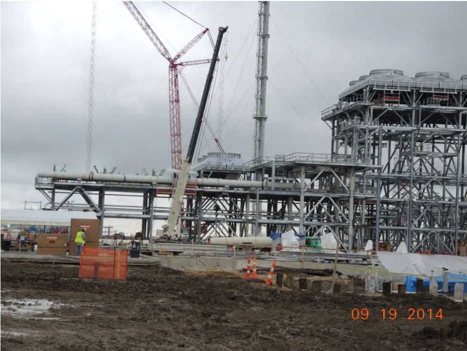
Train 3 Installing Pipe in Propane Rack
