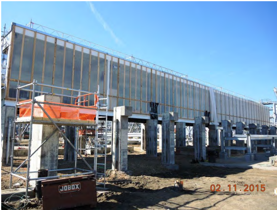
Stage 2 OSBL Utility Substation Area – Setting substation building.
