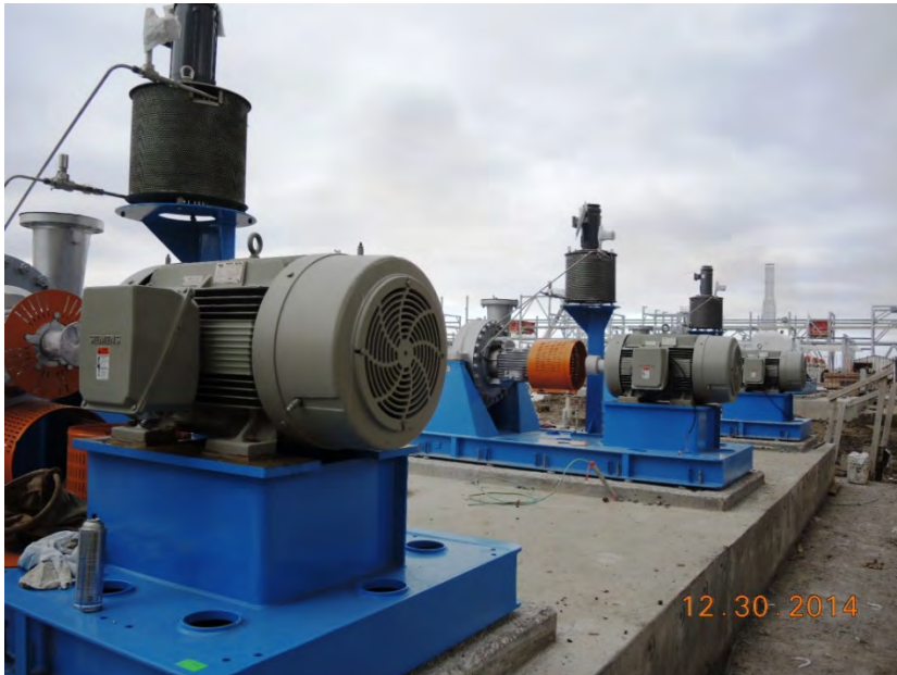
Train 3 Lean Booster Pumps Installed
