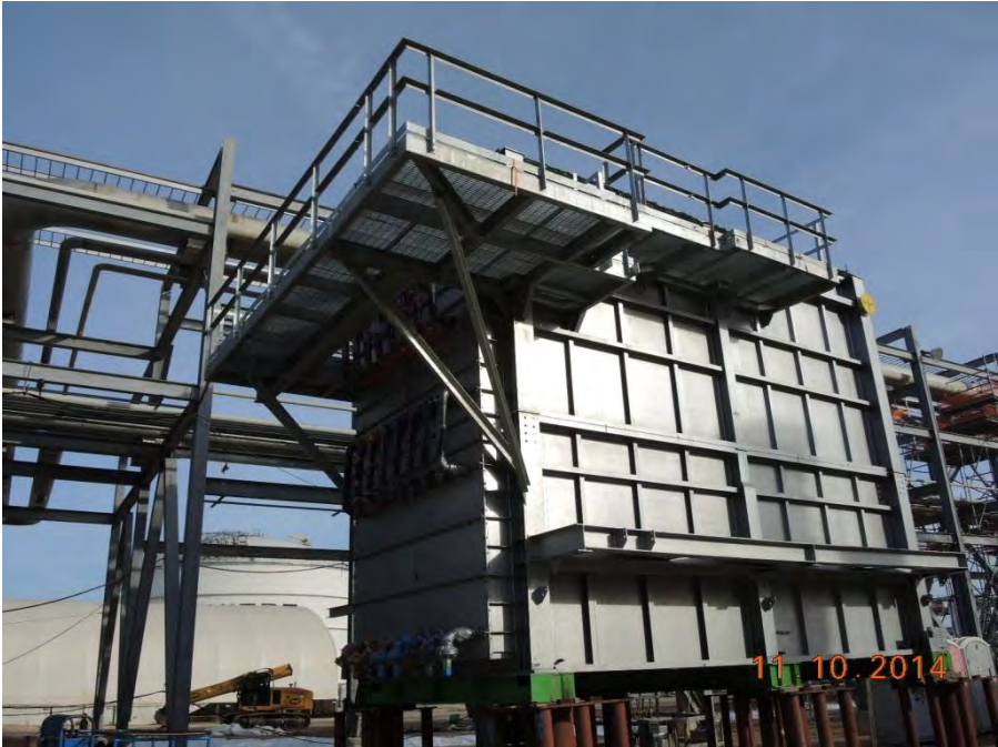
Train 1 Installing Platforms on WHRU
