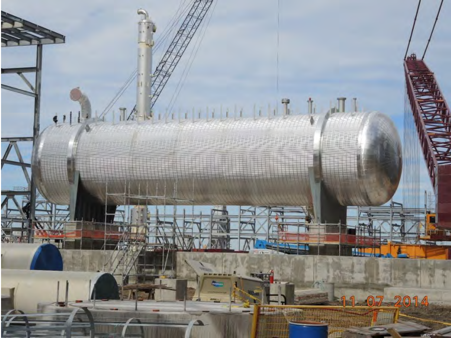
Train 3 Installed Hot Oil Drum
