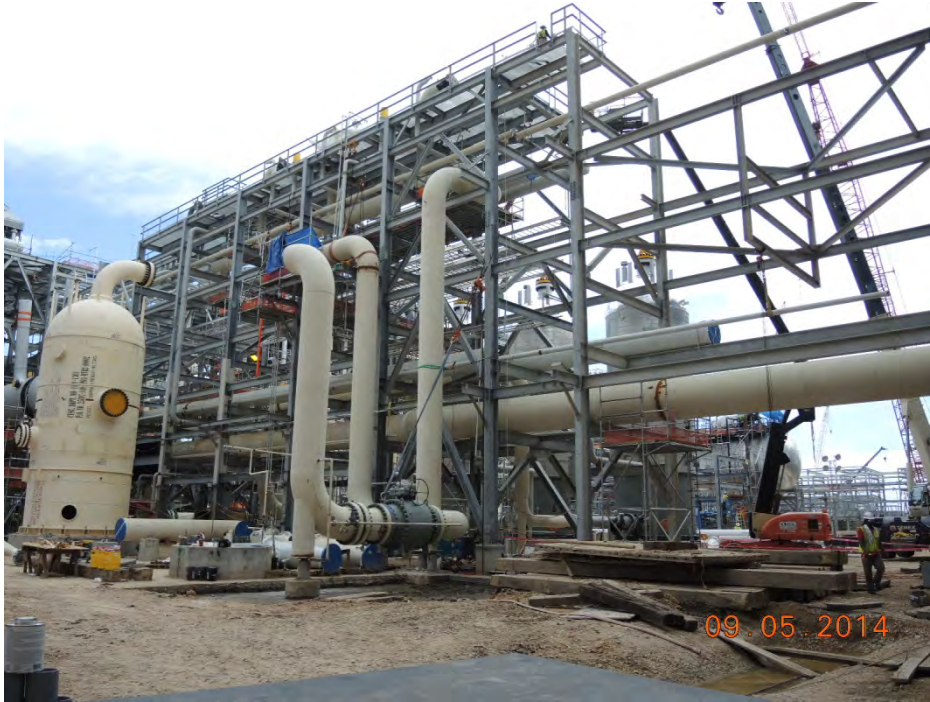
Train 1 Installing Pipe
