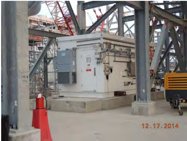
Train 3 Analyzer Shelter
