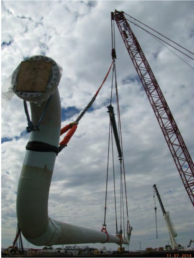
OSBL Stage 1 Pipe Lift
