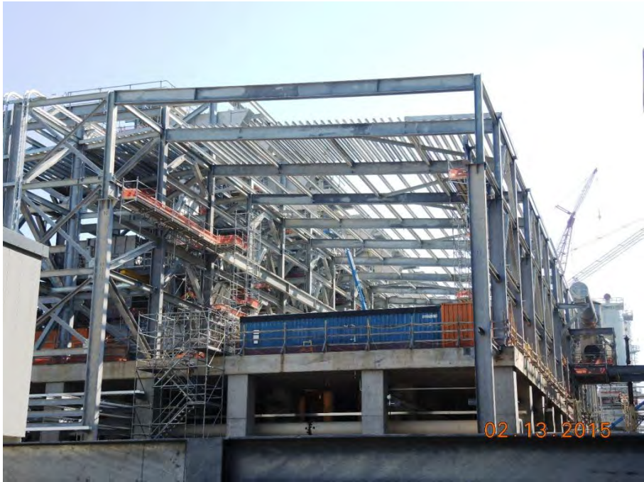
Train 2 Compressor Area – Installing perlins.
