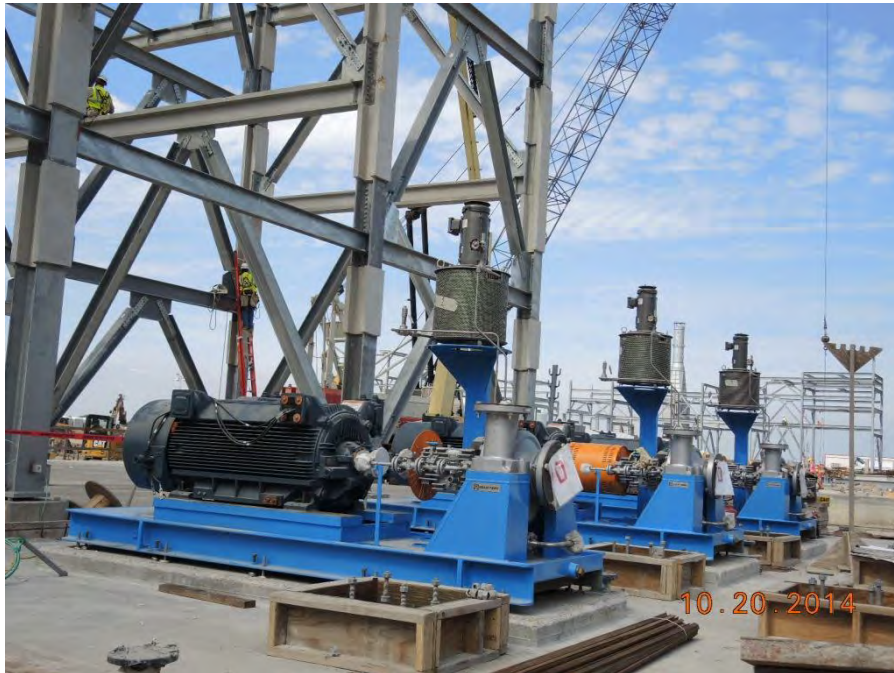
Train 3 Installed Hot Oil Pumps
