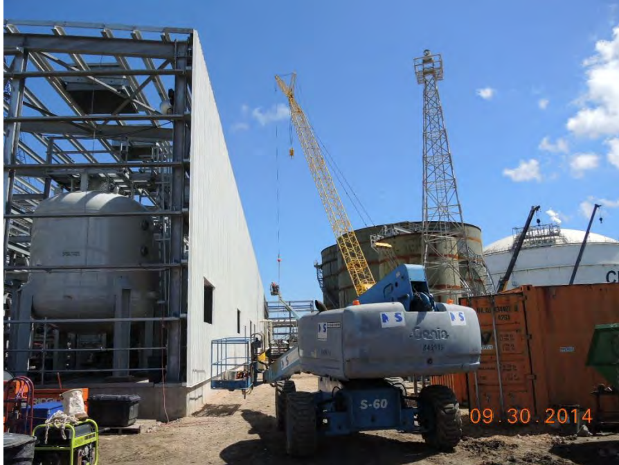
OSBL Stage 1 Installing Siding on Water Treatment Building
