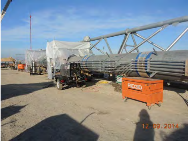
OSBL Stage 2 Start Setting Mechanical Equipment Wet/Dry Gas Flare
