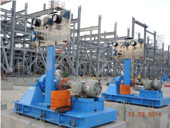
Train 4 Debutanizer Reflux Pumps Installed
