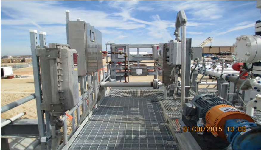
Condensate Storage & Send-Out System – Leased Access Control Transfer (LACT) Skid.
