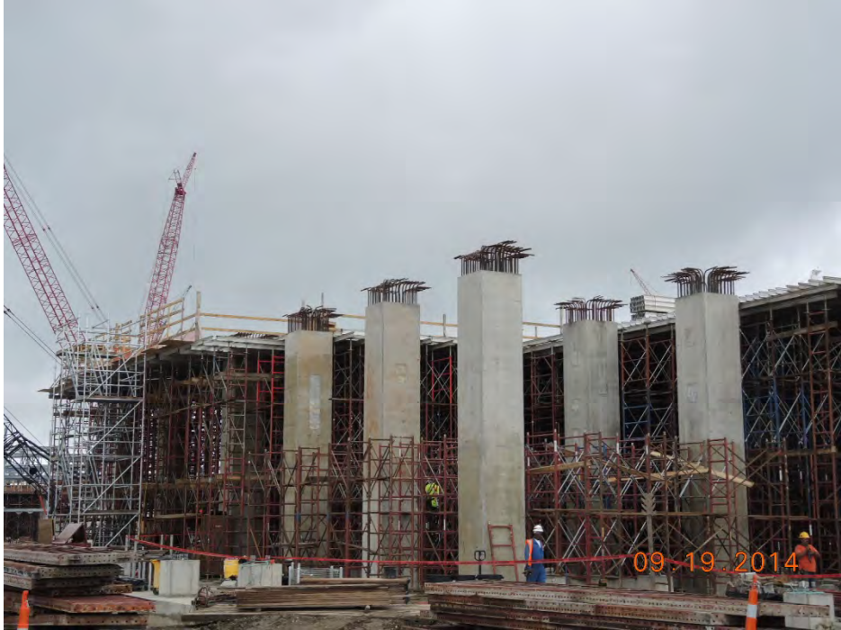
Train 4 Starting form work on Compressor Deck
