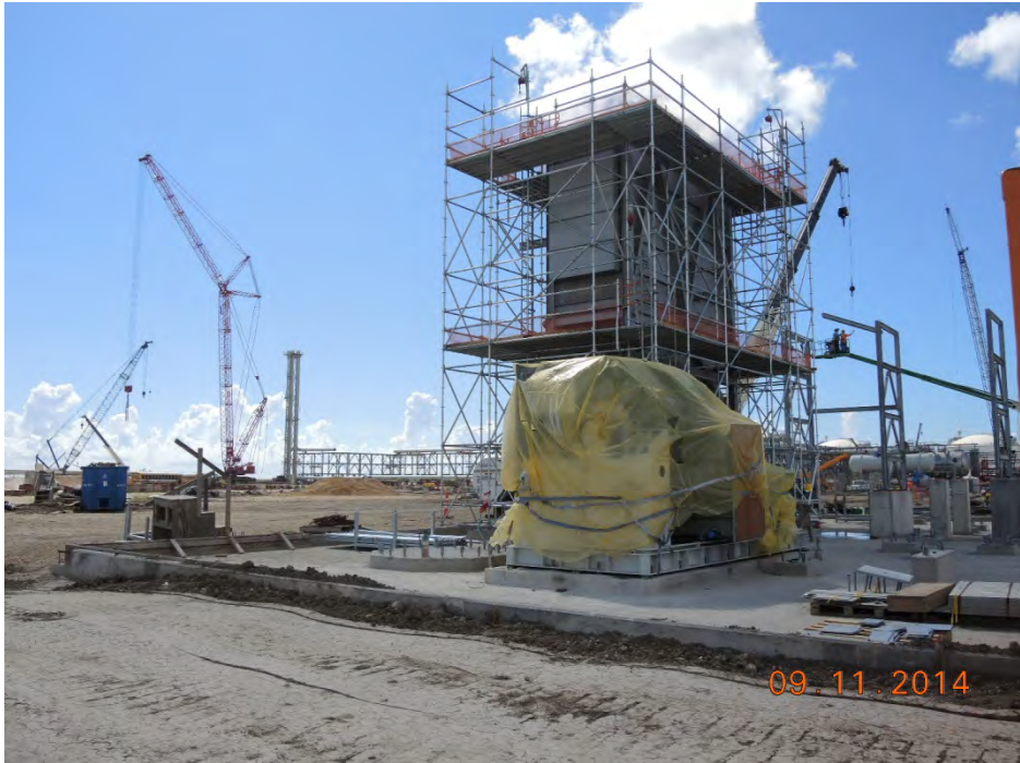
OSBL2 Installed Thermal Oxidizer Fans
