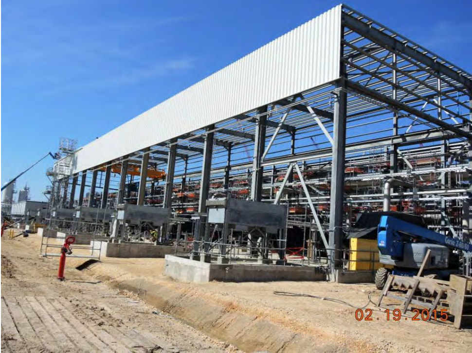
Stage 1 OSBL BOG Compressor Area – Installing siding.
