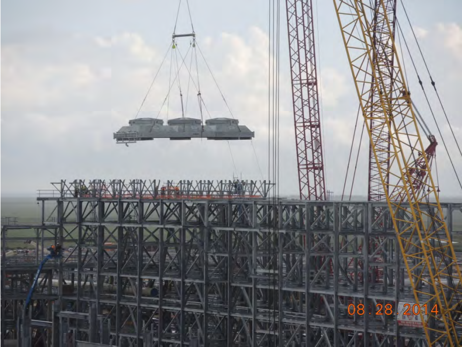
Train 3 Installing Propane Coolers
