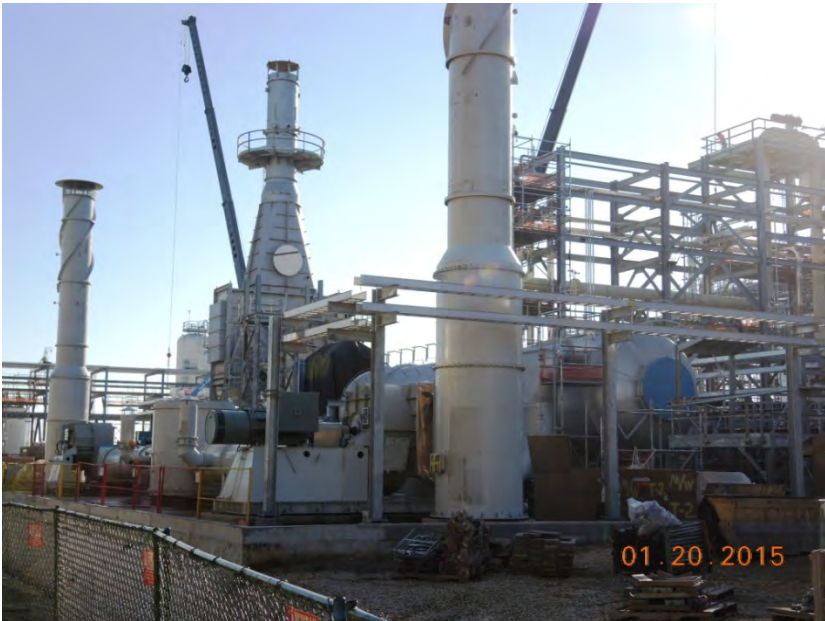
Train 2 Installing Cable Tray around Thermal Oxidizer
