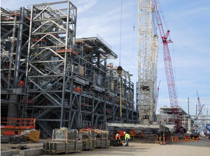
Train 1 Installing Elevated Steel
