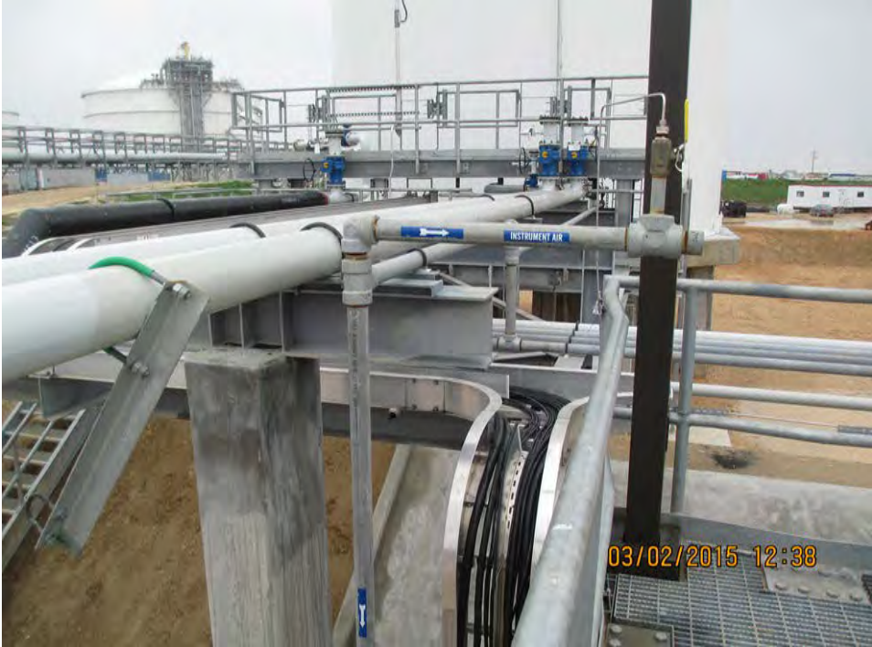
Line labels for instrument air at condensate area.
