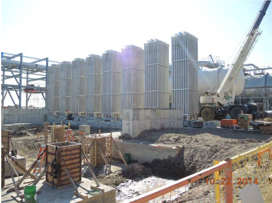
OSBL Stage 2 Installing Dry Gas Flare Vaporizers
