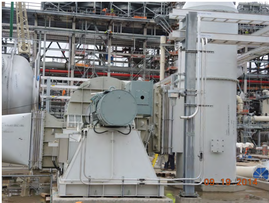
Train 1 Running Electrical Conduit to the Thermal Oxidizer Fans
