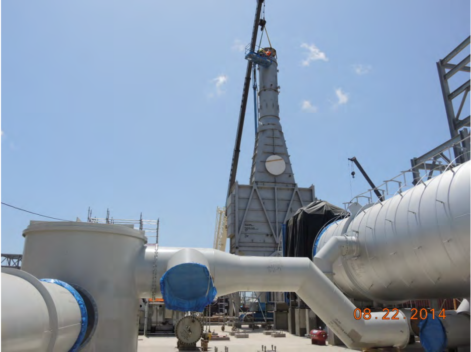
Train 2 Set LS Propane-Ethylene Condensate Feed Chiller
