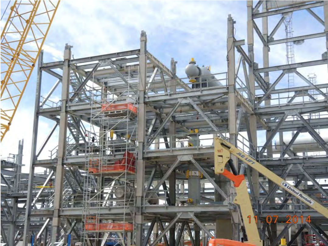
Train 3 Setting Equipment with Steel Installation
