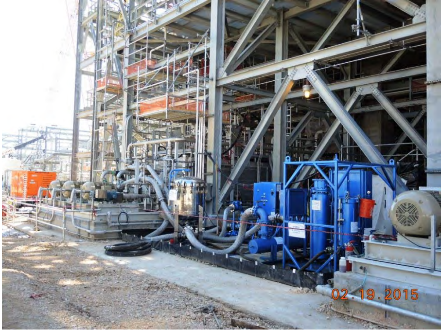
Train 1 Compressor Area - lube oil flush.
