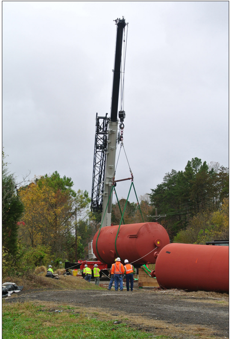
Abandoned tanks at the Y-12 Complex
