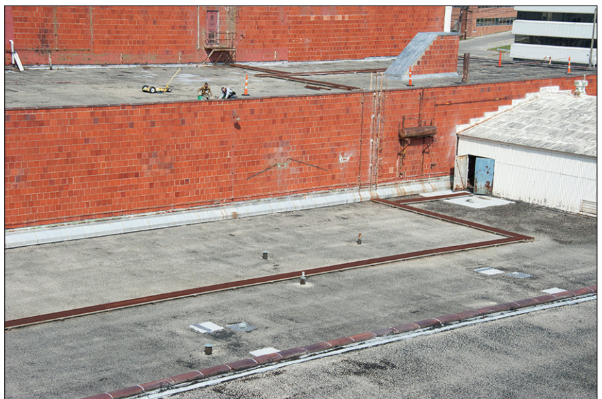
Alpha 4 roof repairs
