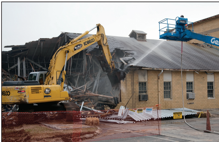
Building 9735 has been demolished.
