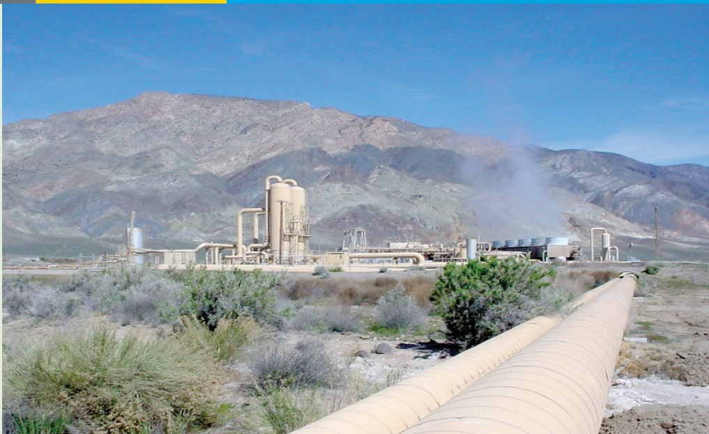
Dixie Valley Bottoming Binary Plant: Terra-Gen was funded by the American Recovery and Reinvestment Act of 2009 to demonstrate the technical and economic feasibility of electricity generation from nonconventional geothermal resources of 223°F, employing the first commercial use of a supercritical cycle at a geothermal power plant inlet temperature of less than 300°F. Since September 2012, the plant has been online and producing 6 MW gross.
