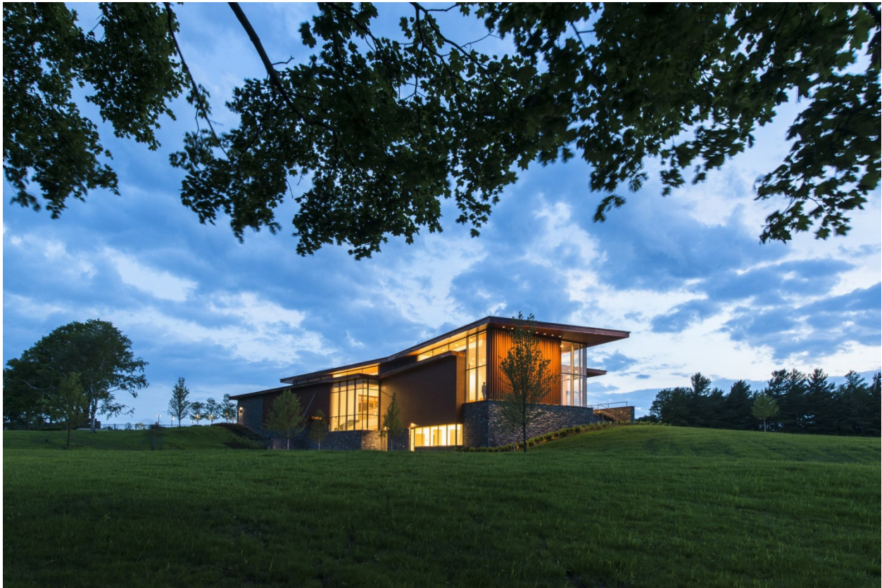
Figure 15 Pizzagalli Center for Art and Education, Shelburne Museum, Shelburne, VT – see Appendix E for more information on the museum's conversion to SSL and difficulty with controls (©Shelburne Museum 2013).
