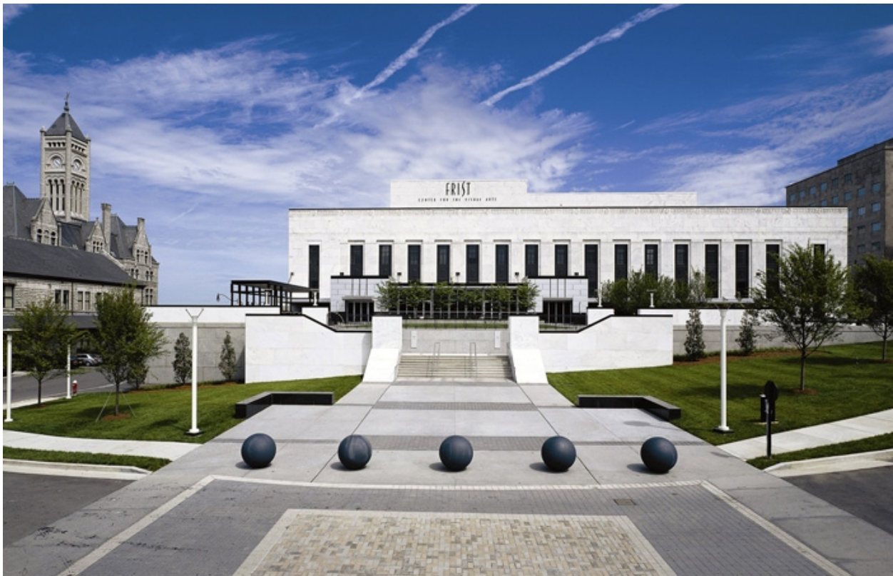
Figure 13 Frist Center for the Visual Arts, Nashville, TN – see Appendix E for more information on the museum’s recently completed retrofit to SSL (©Frist Center).
