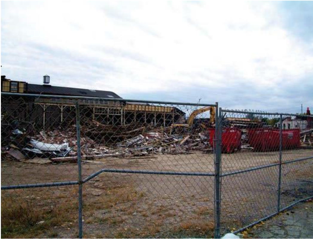
Figure 8. The Site Owner at the Hamilton, Ohio, Site Demolished a Portion of the Remediated Site Building in October 2012
