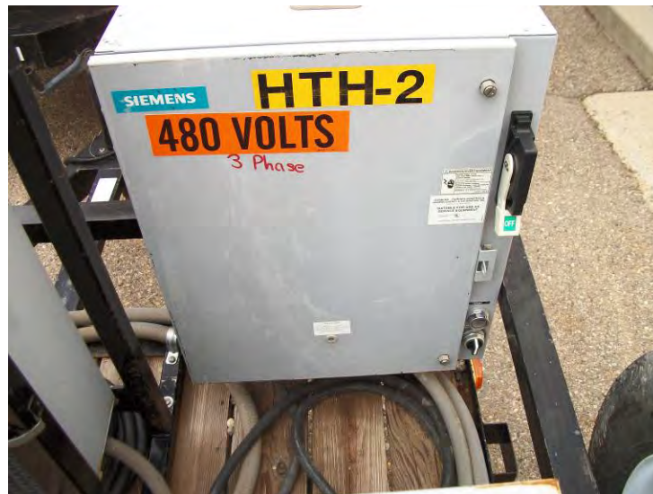
Figure 4. Typical Disconnect Switch
