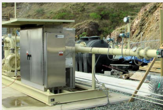
A landfill-gas-to-energy conversion system at Bovoni Landfill on St. Thomas will bring the USVI one step closer to meeting its clean energy goal. Photo from Don Buchanan, VIEO, NREL 20817
