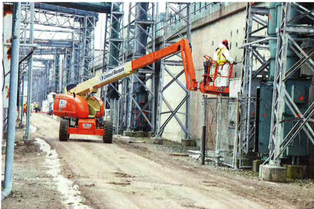
Figure A-12. ACM abatement of X-533B Switch Gear House, looking southeast – March 2010
