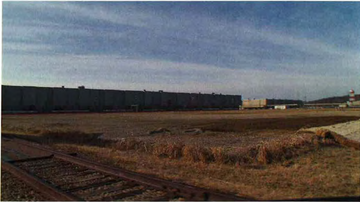
Figure A-22. Location of the former X-533 Switchyard Complex (foreground), looking southwest February 2011
