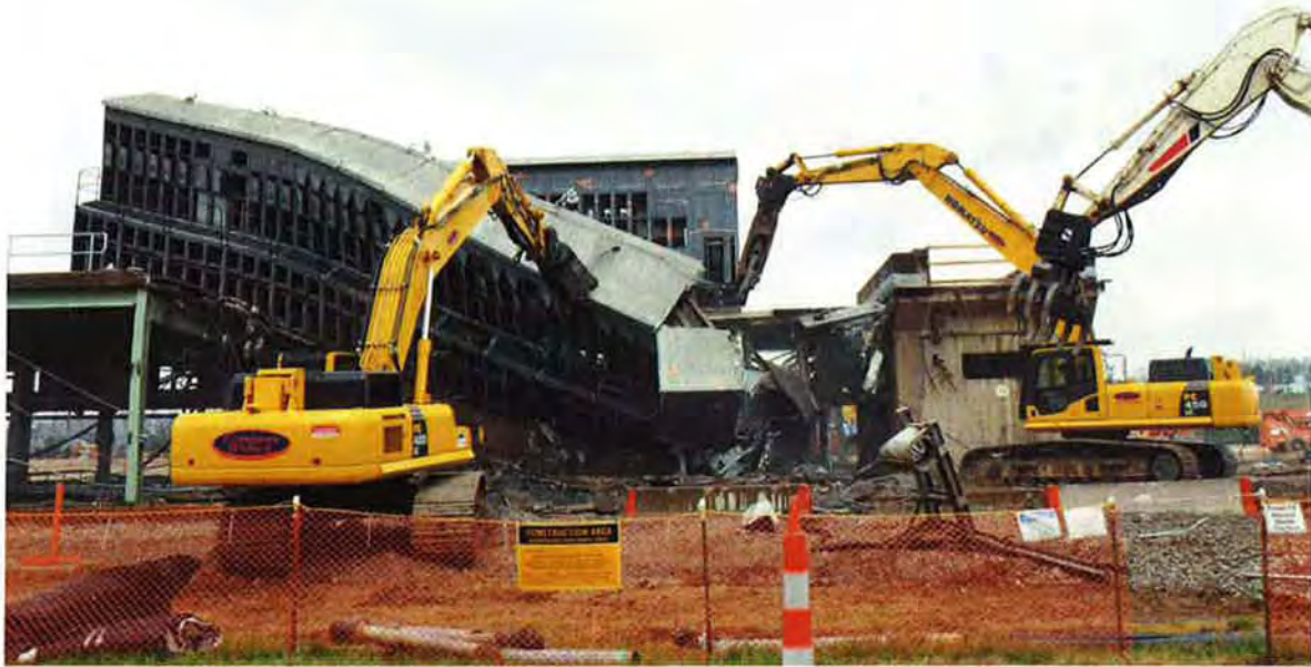
Figure A-17. Removal of X-533B East Switch Gear House electrical cabinets, looking north – November 2010
