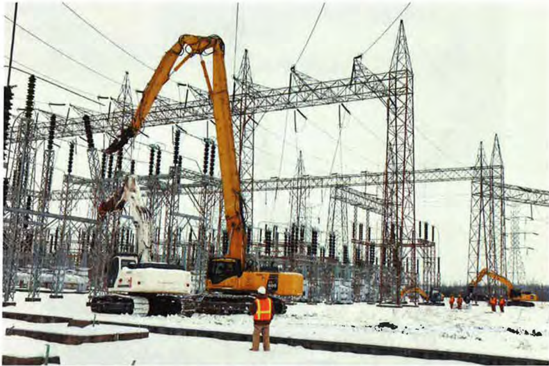
Figure A-11. Demolition of X-533A Switchyard towers – February 2010
