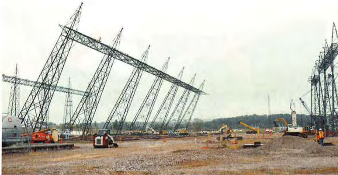
Figure A-15. Demolition of X-533A Switchyard towers, looking east – September 2010
