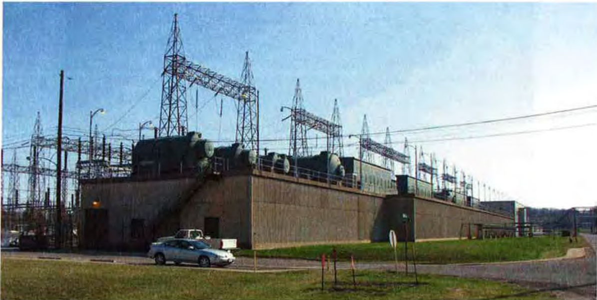
Figure A-4. X-533B West Switch Gear House before demolition, looking northeast – March 2009
