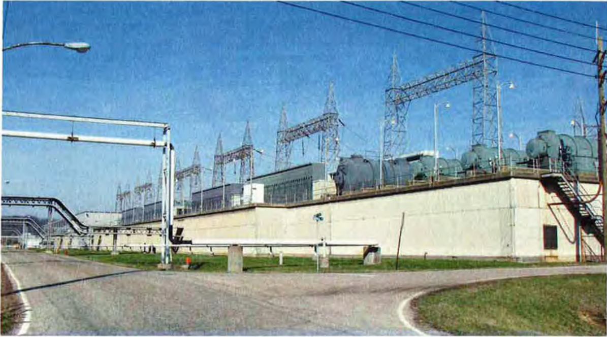
Figure A-3. X-533B East Switch Gear House before demolition, looking northwest – March 2009
