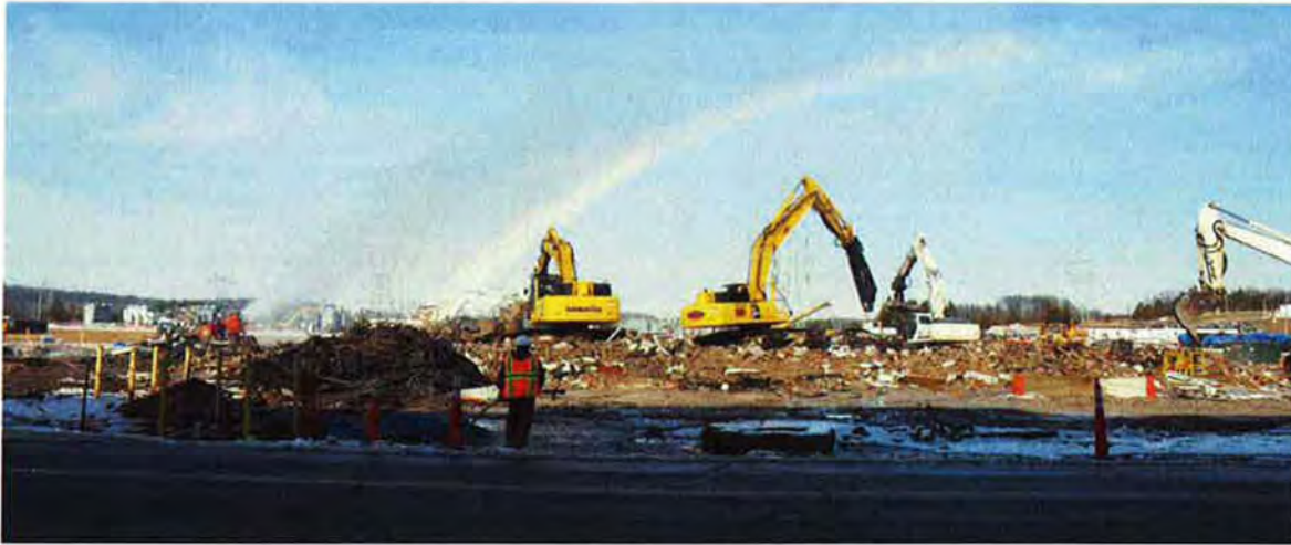
Figure A-19. Loading of debris from X-533B Control Room, looking north – December 2010
