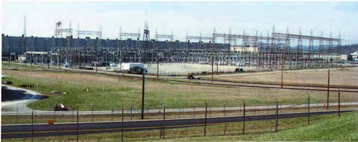
Figure A-1. X-533 Switchyard Complex before demolition, looking southwest – March 2009
