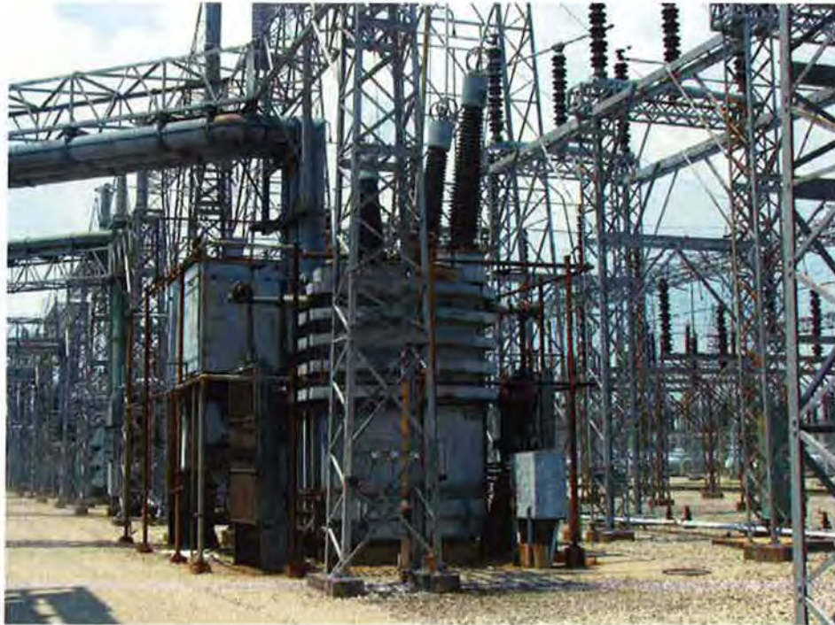
Figure A-9. Power transformer in the X-533A Switchyard before demolition, looking northwest – June 2009
