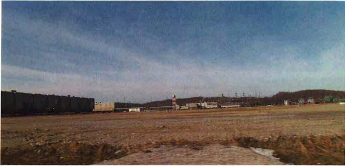
Figure A-21. Location of the former X-533 Switchyard Complex (foreground), looking west February 2011
