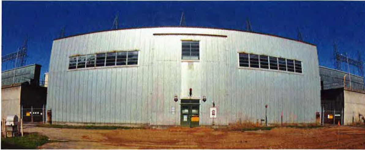
Figure A-5. X-533B Control Room before demolition, looking north – December 2009
