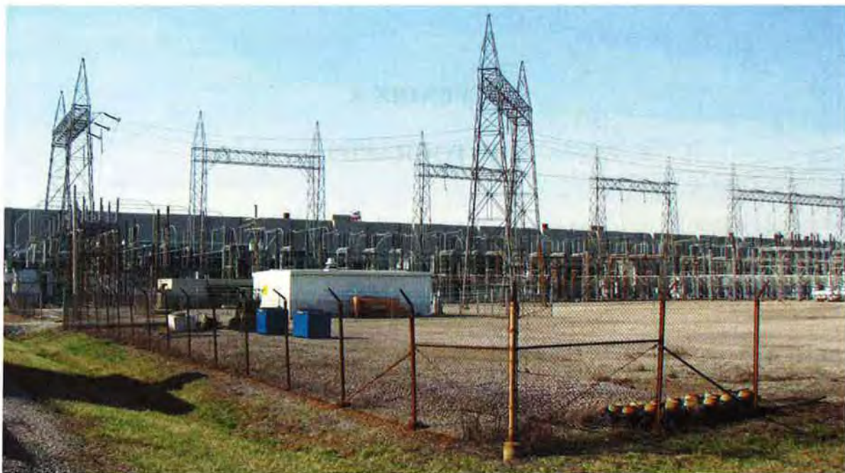
Figure A-2. X-533 Switchyard Complex before demolition, looking southwest – March 2009
