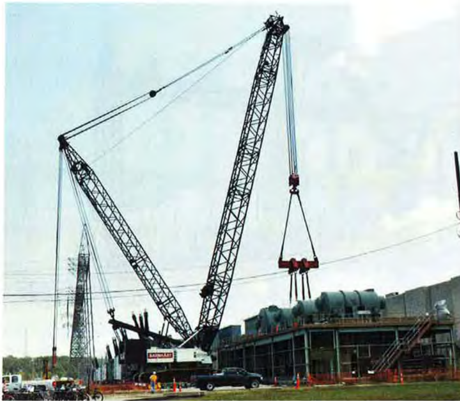
Figure A-13. Removal of synchronous condensers from X-533B West Switch Gear House, looking southeast August 2010
