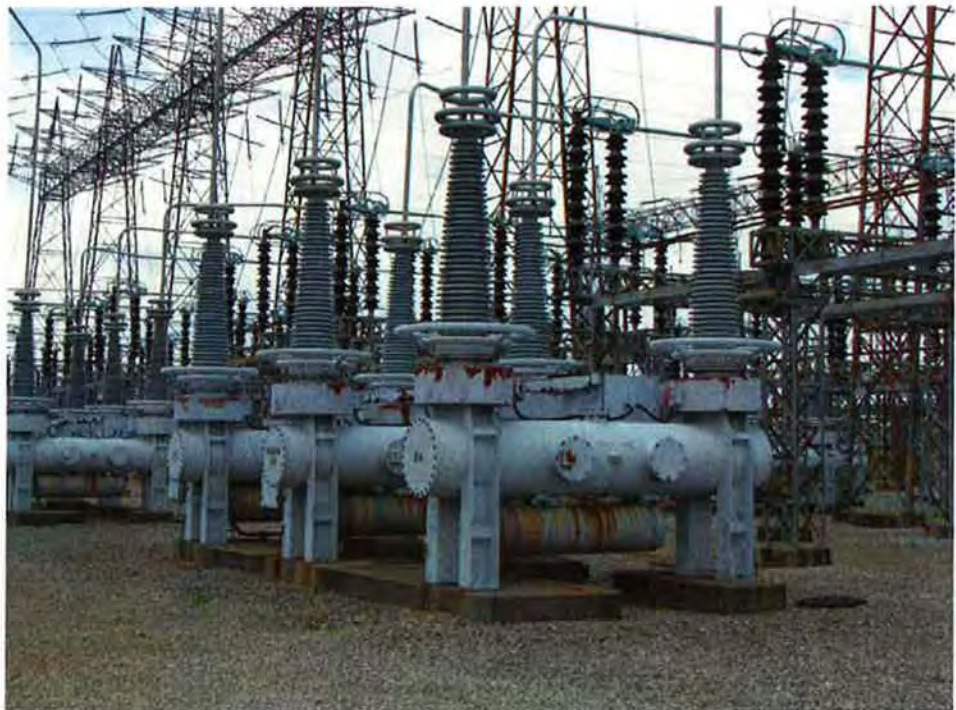
Figure A-8. Gas circuit breakers before demolition – June 2009
