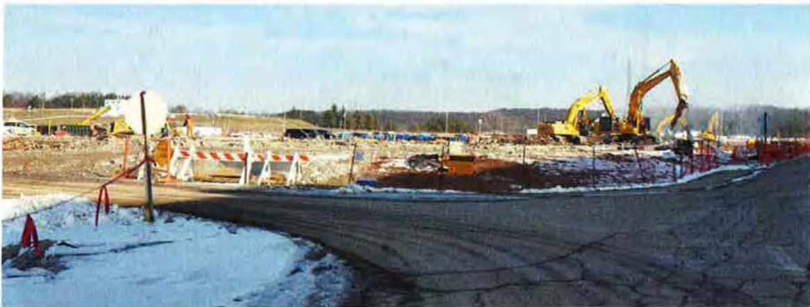
Figure A-18. Loading of debris from X-533B West Switch Gear House, looking east – December 2010
