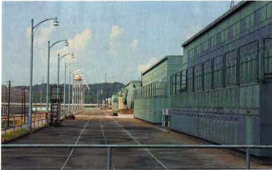
Figure A-7. Electrical cabinets on top of X-533B Switch Gear House roof before demolition, looking west August 2009
