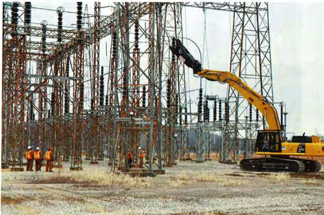
Figure A-10. Demolition of X-533A Switchyard towers – February 2010
