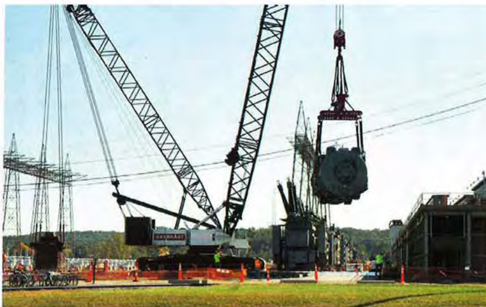
Figure A-14. Removal of synchronous condenser from X-533B West Switch Gear House, looking east September 2010
