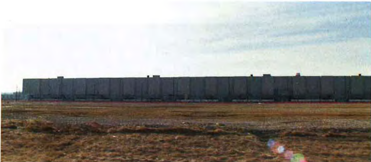
Figure A-20. Location of the former X-533 Switchyard Complex (foreground), looking south February 2011
