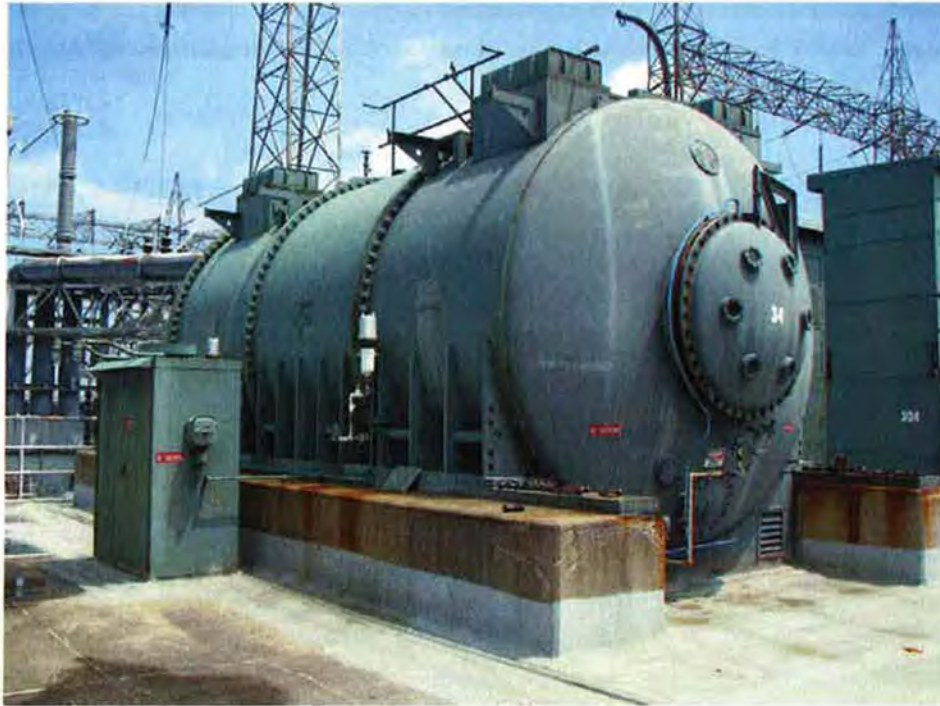
Figure A-6. Synchronous condenser mounted to X-533B Switch Gear House roof before demolition June 2009
