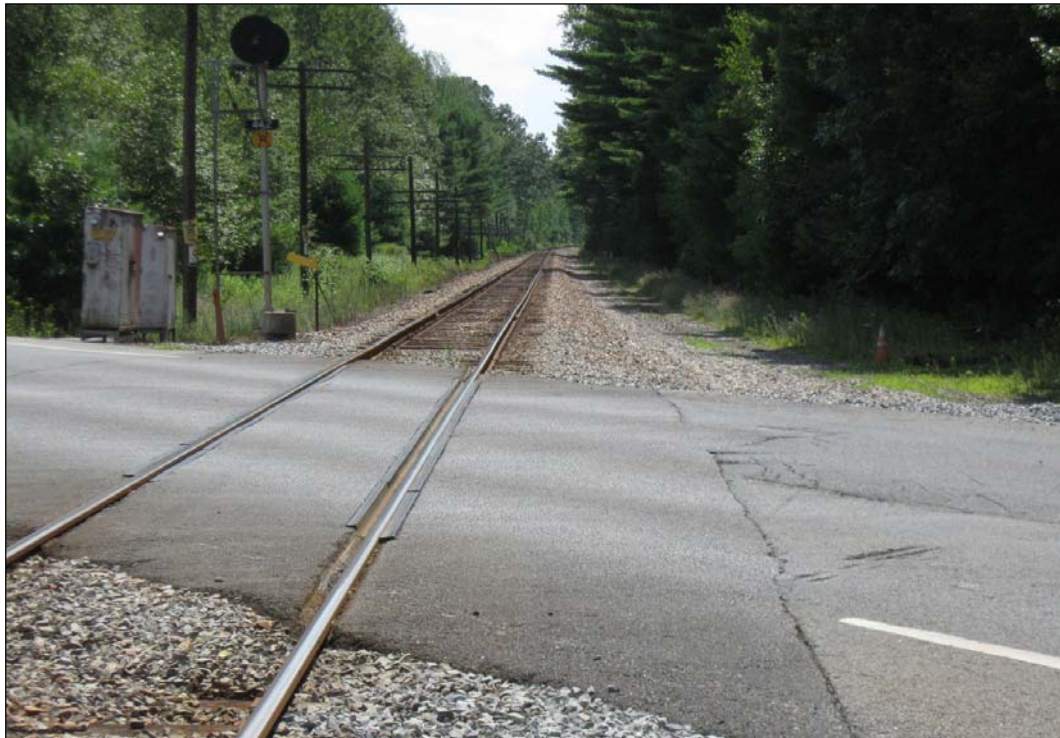
Note: This photograph shows a southwest view of the location of a proposed cooling station near MP 146. The cooling station would be visible on the west (right) side of the railroad tracks.
