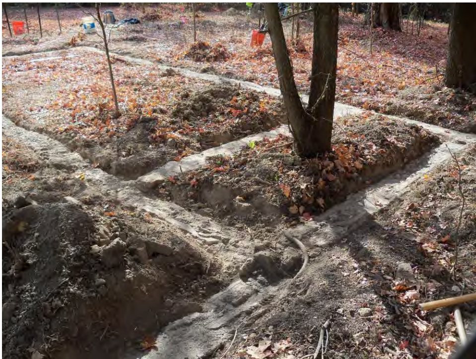
Plate 2. House foundation at 33PK184; facing southwest.
