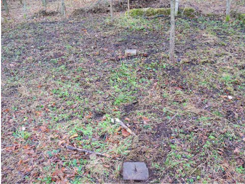
Plate 69. Barn foundation at 33PK197 showing the internal foundation piers in line with the south edges of the barn door openings; facing southeast.
