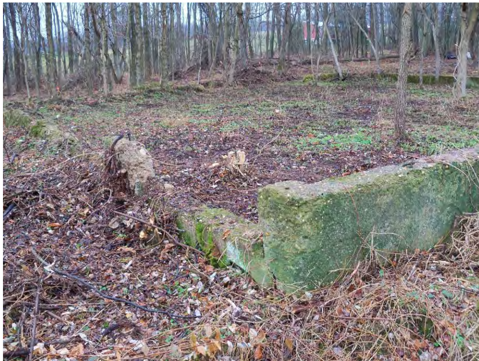
Plate 68. Barn foundation at 33PK197 showing the pedestrian door opening in the north corner; facing south.
