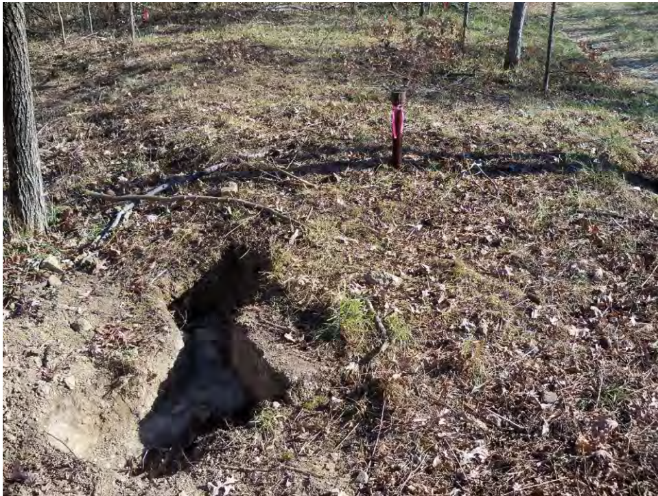
Plate 42. Southeast corner of Building 4 at 33 PK194 showing the raised area of concrete; facing southeast.
