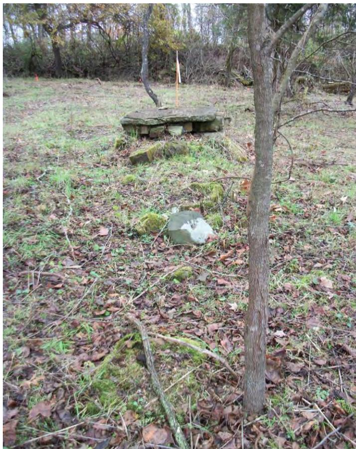
Plate 4. Collapsed stone-pier foundation along the east edge of the house at 33PK322; facing northeast.
