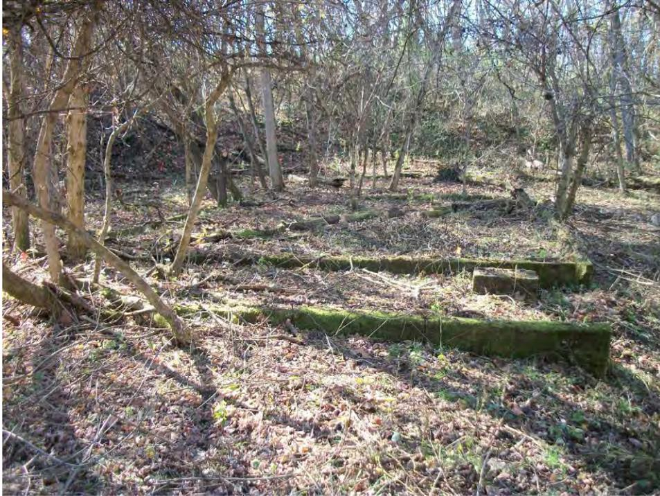
Plate 23. Floor of Barn 3 foundation remnant showing interior walls and machine pad; facing west-southwest.
