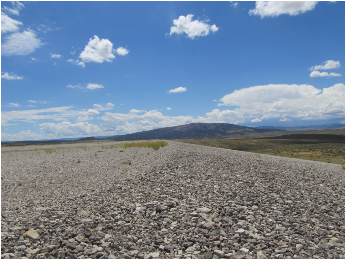
MAW 8/2014. PL-8. Intersection of west side slope and top of disposal cell.
