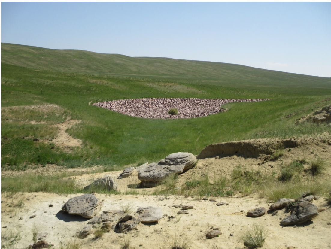
SBS 7/2014. PL-8. Outlet of riprap-armored drainage channel.
