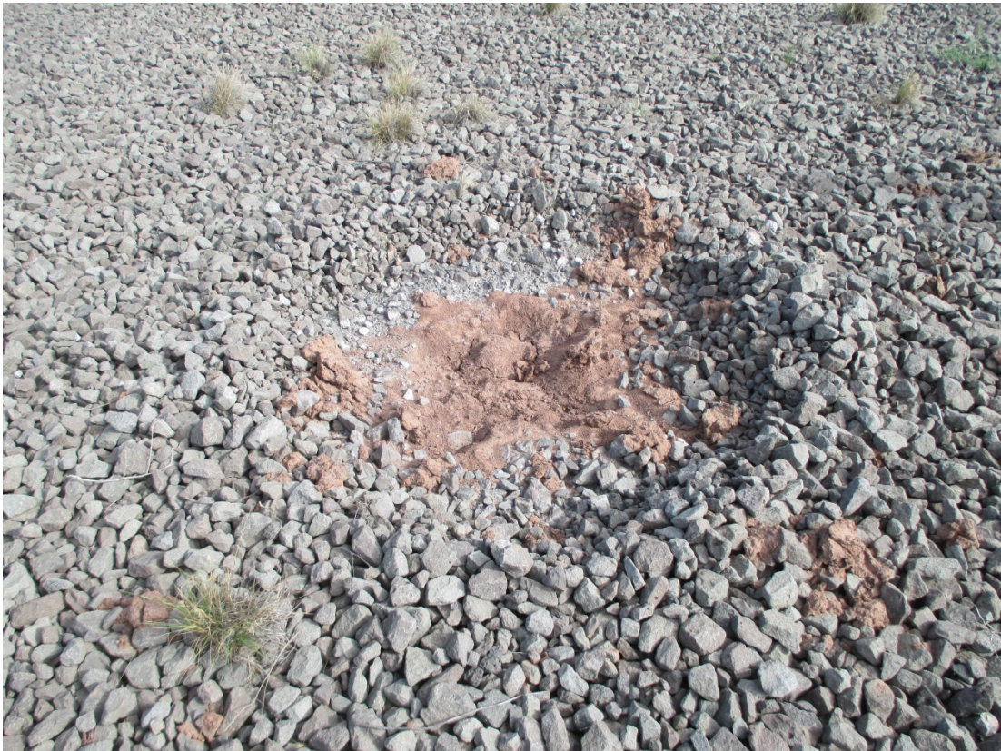
BLU 8/2014. PL-10. Exposed radon barrier surface on carbonate tailings disposal cell top slope.
