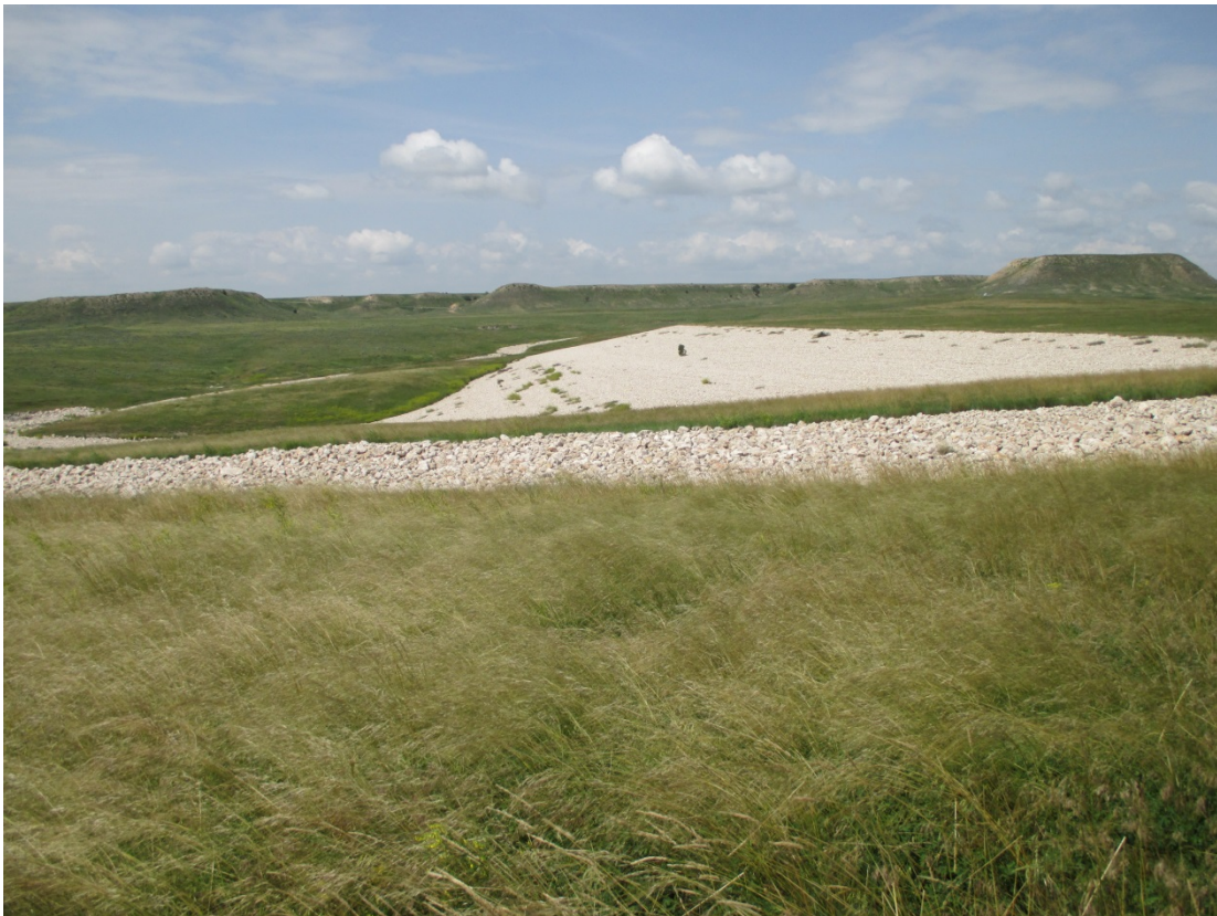
EDG 7/2014. PL-5. View west across tailings embankment.
