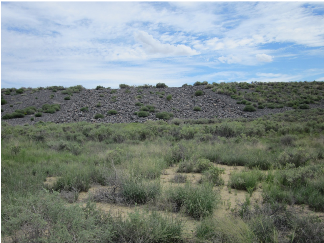
BAR 8/2014. PL-6. Rock-armored tailings impoundment spillway.
