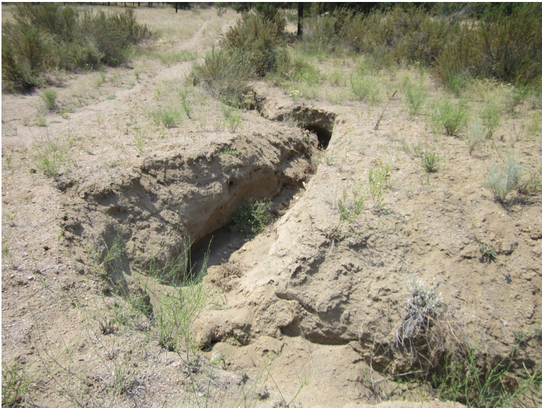
SHE 7/2014. PL-4. Erosion near perimeter sign P2.
