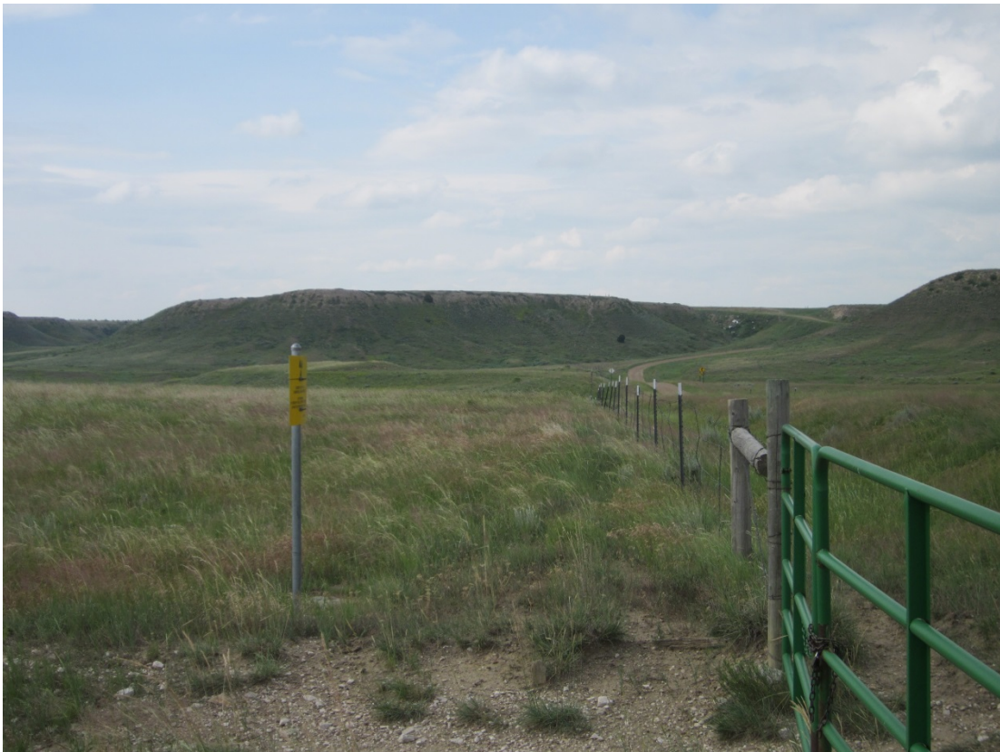
EDG 7/2014. PL-1. Site entrance gate and sign.
