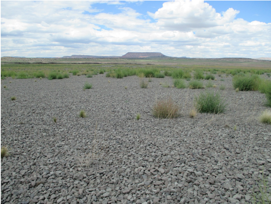
BLU 8/2014. PL-7. Vegetation on main tailings disposal cell top slope.
