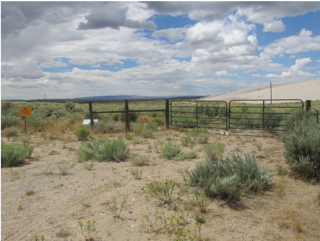
MAW 8/2014. PL-1. Entrance gate, entrance sign, and site marker (disposal cell in background).
