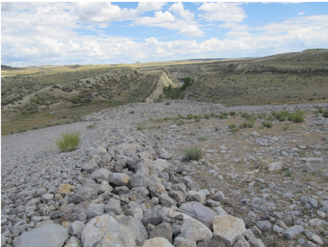
MAW 8/2014. PL-6. Diversion Channel No. 1 outlet into launch rock erosion protection basin on east side slope of disposal cell (Rob Pit in the background).
