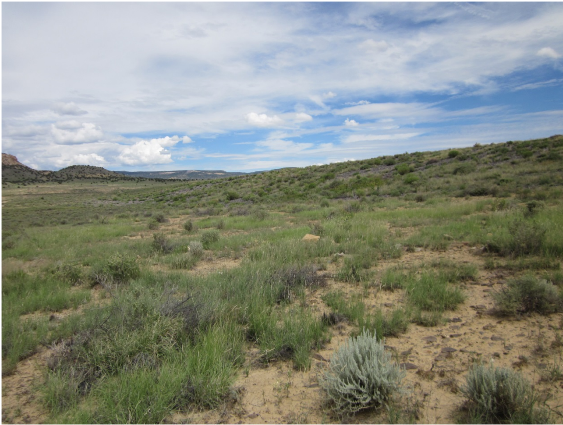
BAR 8/2014. PL-7. Tailings impoundment containment dam.
