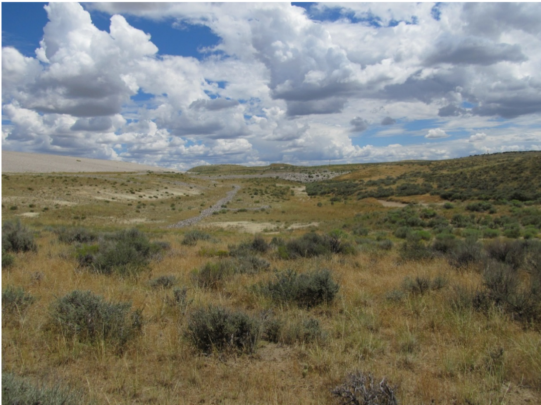
MAW 8/2014. PL-10. Southwest portion of site (Diversion Channel No. 2, ancillary cell, and disposal cell in background).
