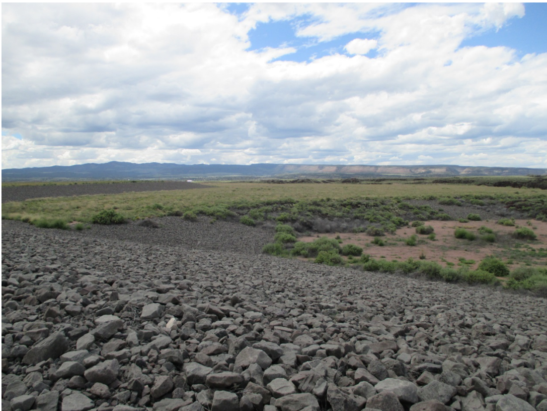
BLU 8/2014. PL-6. Acid tailings disposal area adjacent to main tailings disposal cell.
