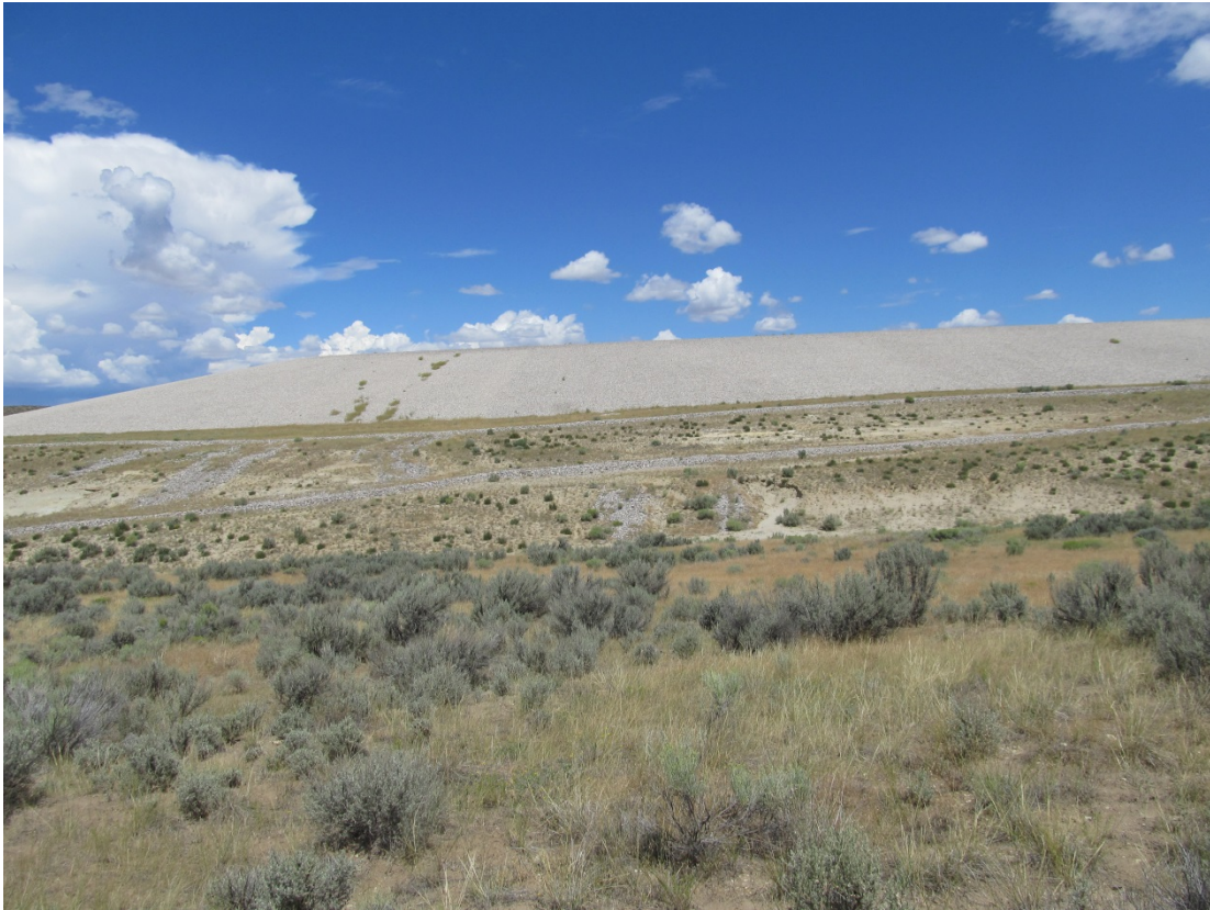
MAW 8/2014. PL-11. Diversion Channel No. 2 (rock berms and southwest portion of disposal cell in background).
