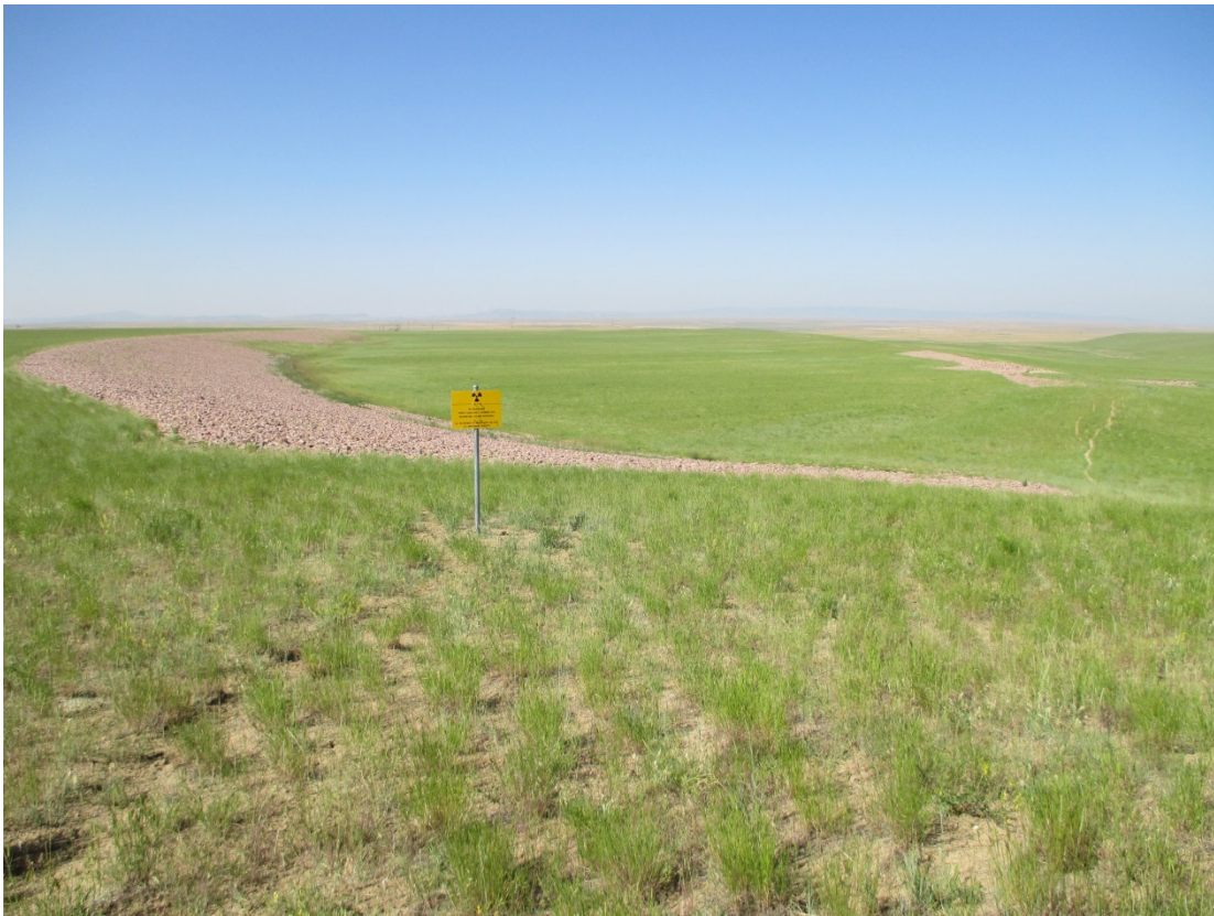
SBS 7/2014. PL-5. Lower surface of disposal cell.
