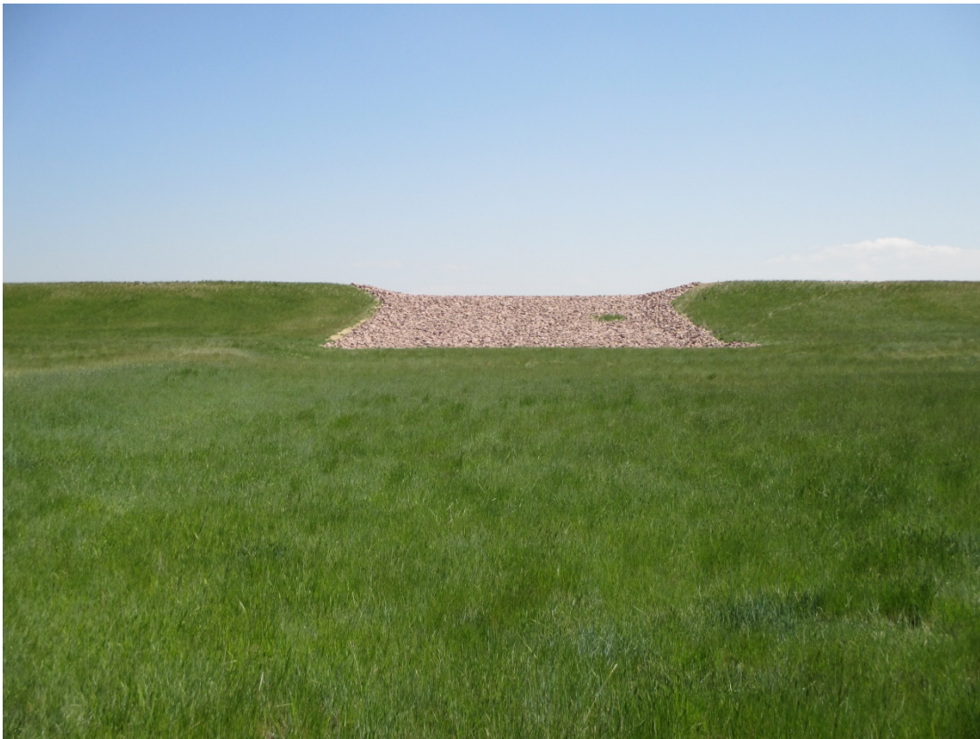
SBS 7/2014. PL-7. South swale discharge point.
