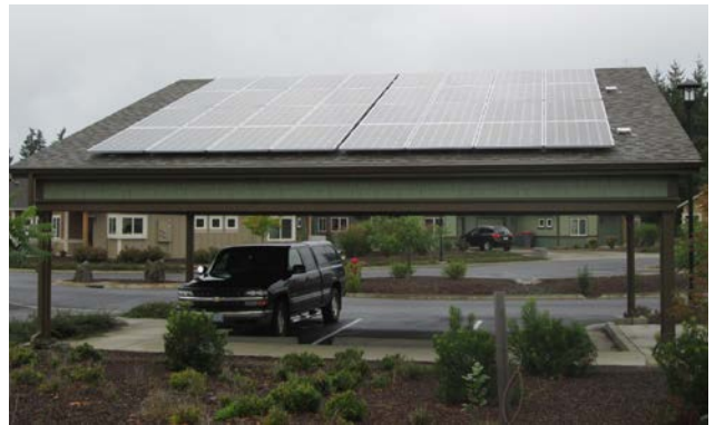
PV panels installed on Grand Ronde Tribal Housing Authority carport. Photo from Grand Ronde Tribal Housing Authority, NREL 31794
