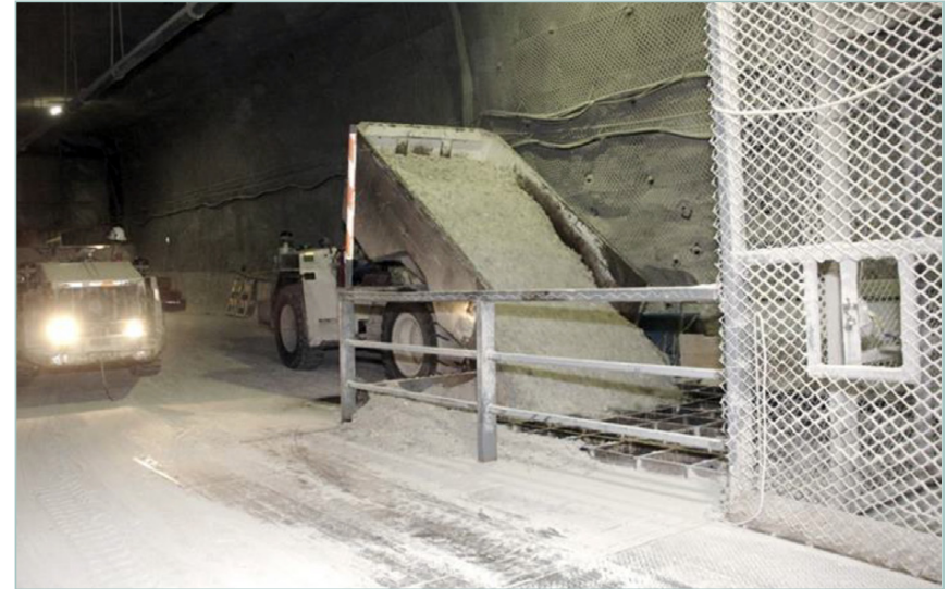
Figure 1-2. Mined salt is dumped at the loading pocket
