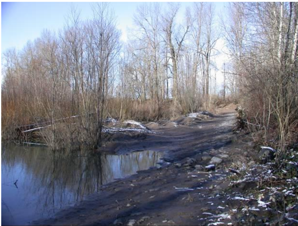
Figure 20 - East Channel dam, to be removed.
