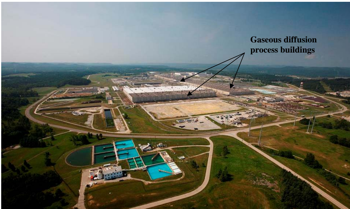
Figure 1.1 The Portsmouth Gaseous Diffusion Plant.
