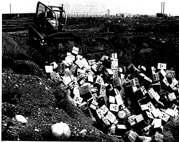
Figure 2-19: Covering and Backfilling Over Filled Trench
