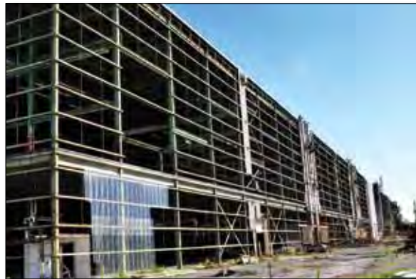
After all the transite panels were removed demolition on the K-31 Building at ETTP began in early October.
