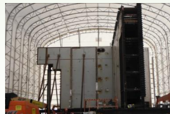
Completed Unit 2 CA05 module and progress on Unit 3 turbine building (Courtesy of SCANA)
