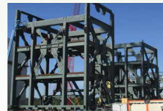
Completed Unit 2 CA05 module and progress on Unit 3 turbine building (Courtesy of SCANA)
